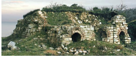
Figure 3: Evcik Church: It has built where the Anastasios Walls meet the Black Sea. The building, which is thought to be a work of the 11th century, is now only a ruin.[18]
