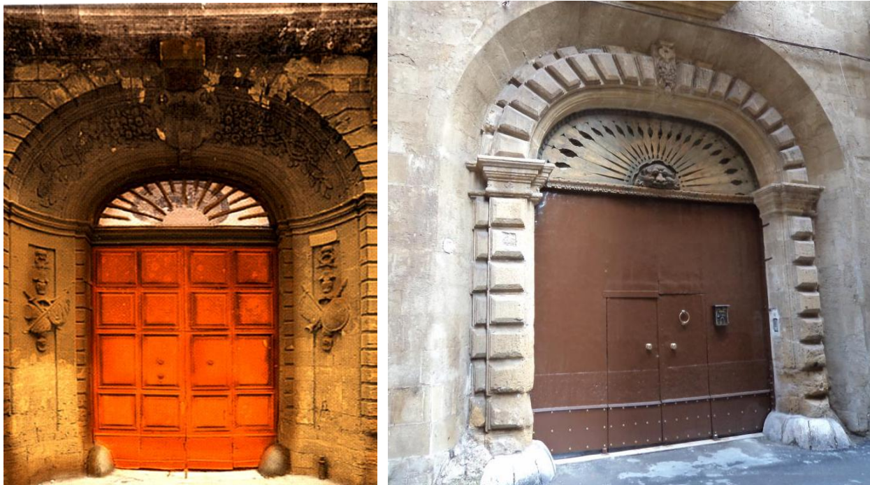
Figure 2: Monumental Portal of Palazzo Ulmo (XVIII sec.) with a stereotomical double-curvature surface, and the Portal of Palazzo de Bellis (XVII sec.) with a rusticated treatment of the stones.
