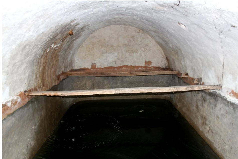
Figure 3: Interior of water cistern space, timber ties, Beja house
