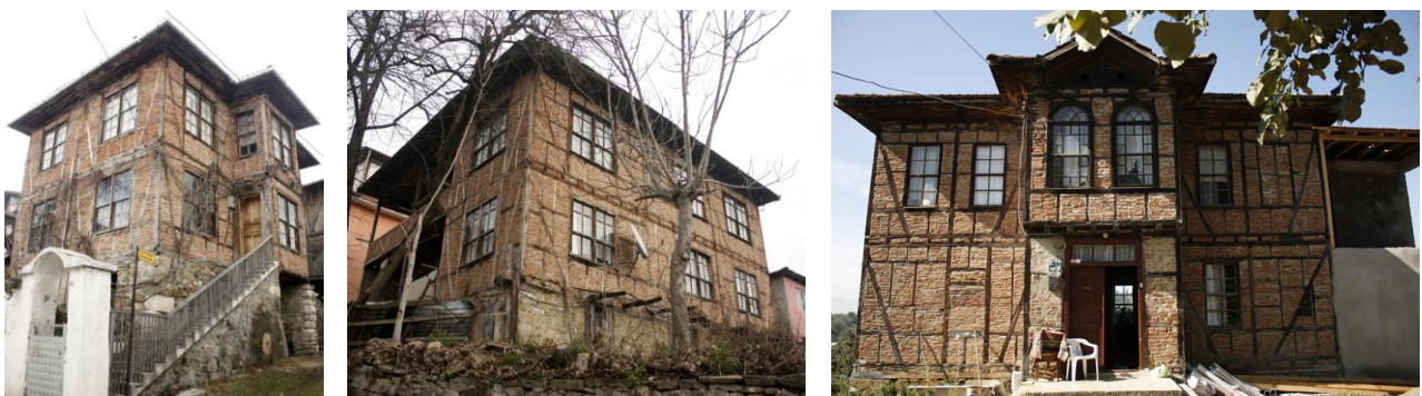
Figure 13: Traditional houses with wooden frame – brick filling system construction (Okur Coşkunçay, 2013)
