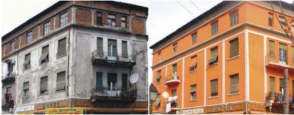
Figure 6: Before and after the repainting
