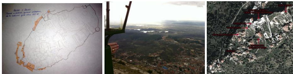
Figure 3: Restorations works, architectural tracking, and cleaning works in Kruja citadel. (Institute of Cultural Monument, Tirana, Albania; K.Xhexhi 2013; Google earth 2013)
