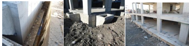
Figure. 3.2.1: The foundation of the project.
