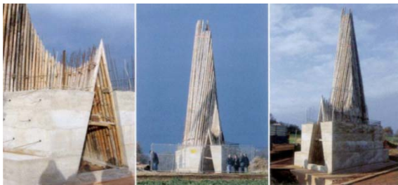
Fig. 5: Zumthor, Bruder Klaus Chapel, constructive process for a massive monolith
