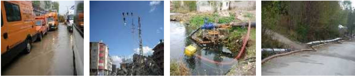
Figure 1. Infrastructure pipeline and energy transfer line damages and the rearranged water transmission lines
