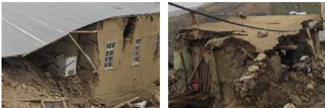
a) March 8, 2010 Elazı -Kovancılar earthquake
