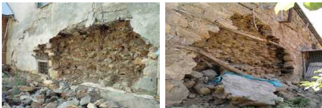
a) March 8, 2010 Elazı -Kovancılar earthquake
