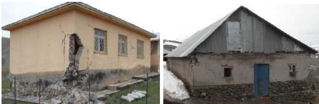
a) March 8, 2010 Elazı -Kovancılar earthquake
