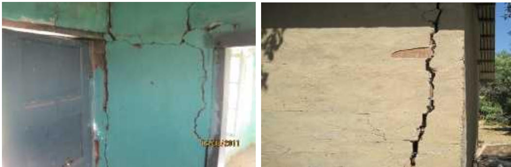
b) June 23, 2011 Elazı -Maden earthquake
