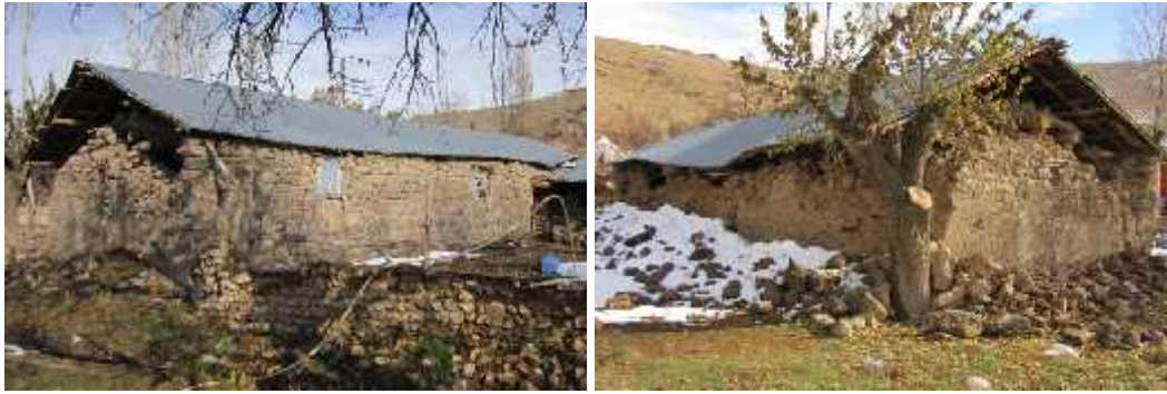
c) 2011 Van earthquakes
