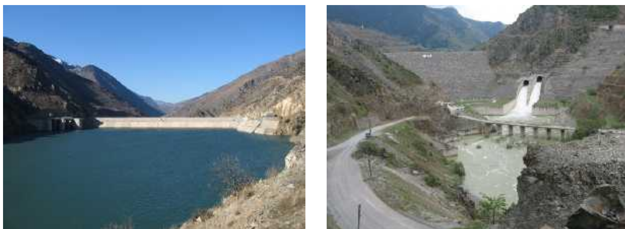
Figure 2 Views of the Kurtun CFRD and its spillway
