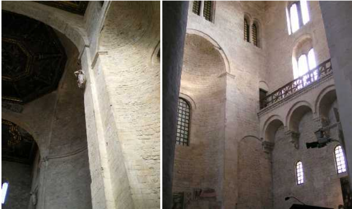
Figure 5 Apsidal facades from the interior
