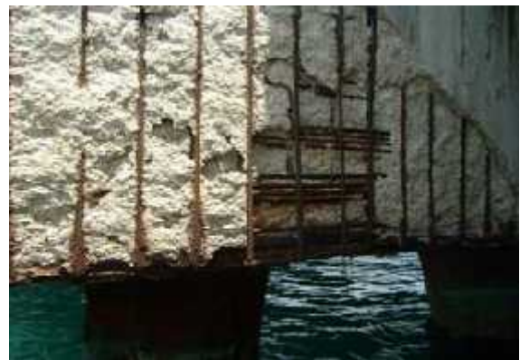
Detachment of concrete cover
