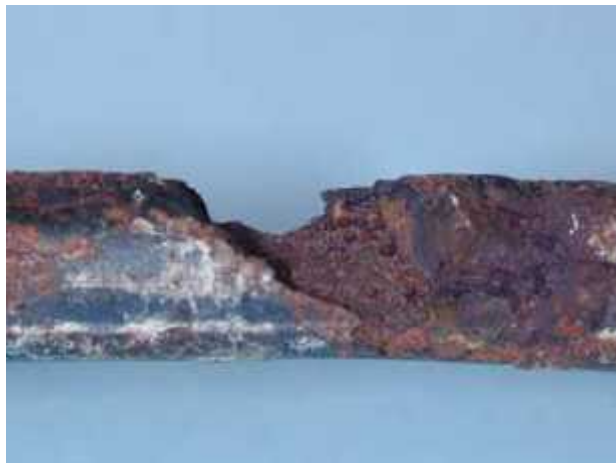
Reduction of cross section of rebar Penetration the of corrosion
