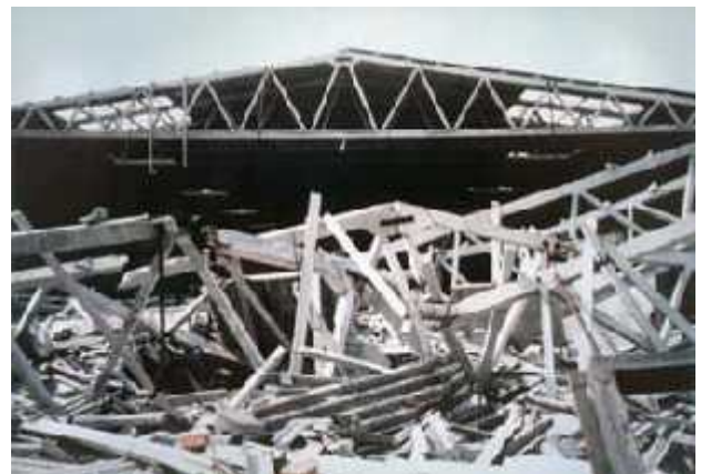
Collapse of the structure Collapse of structur
