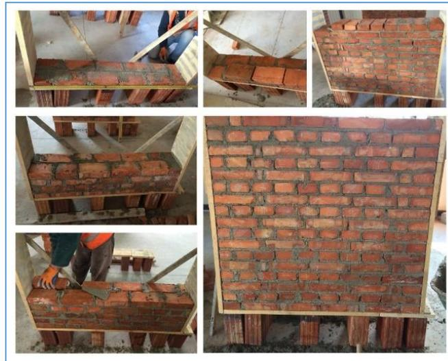
Figure 21. Construction process of plain walls.
