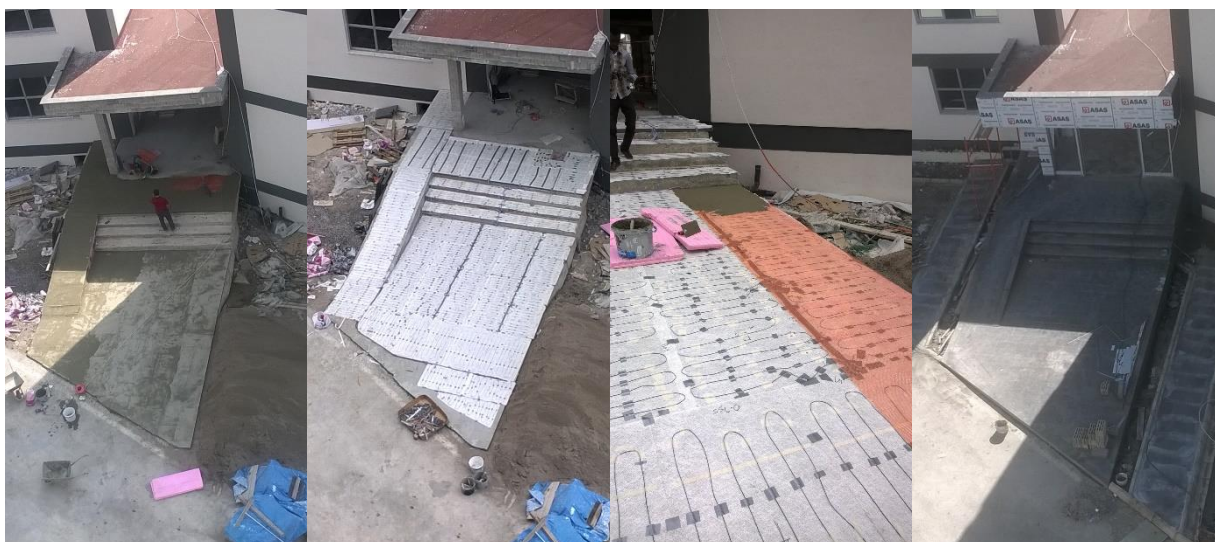
(a) Insulation at the bottom
