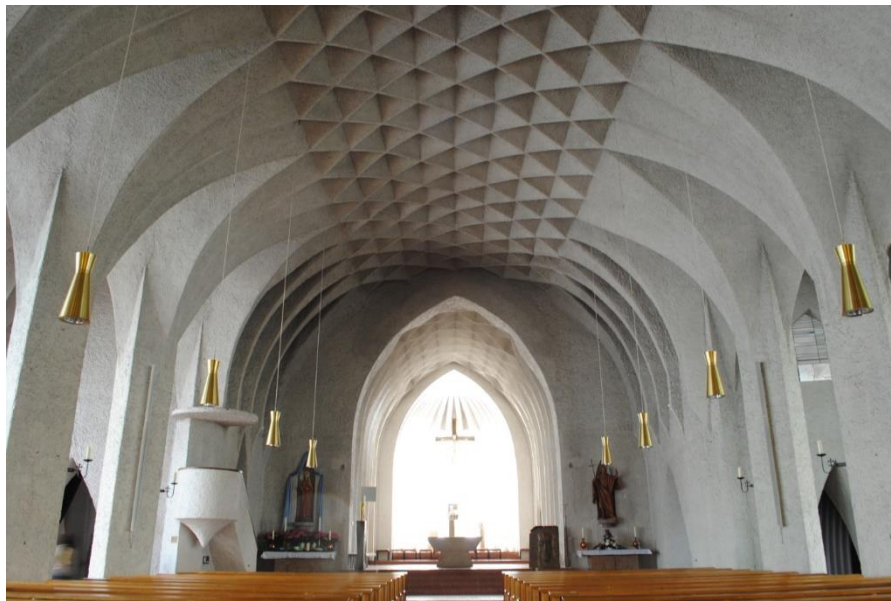
Fig. 5 - Internal view © Giovanni Carbonara (2015)
