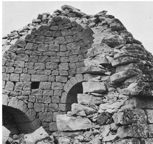
Fig. 3. Example of partial collapse of trullo vault [1]
