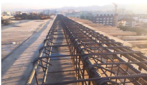
Figure 6. In – Placement of stirrups
