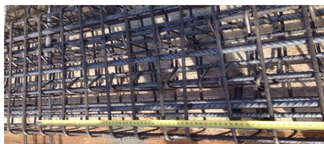
Figure 7. Measurement of spacing between stirrups
