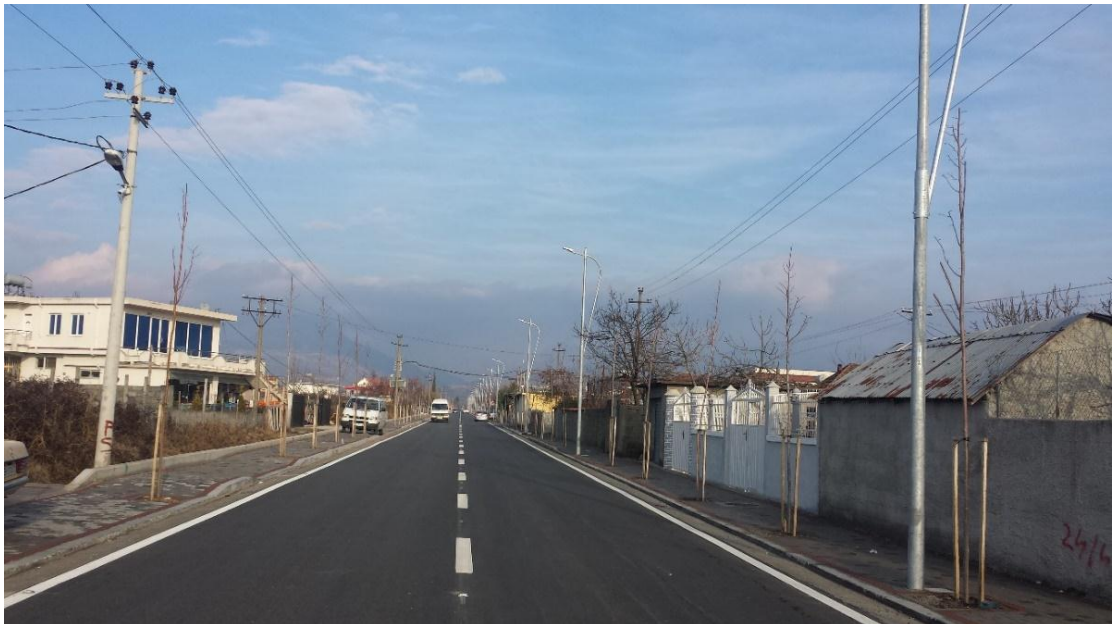
Figure 17. Completed part of the project
