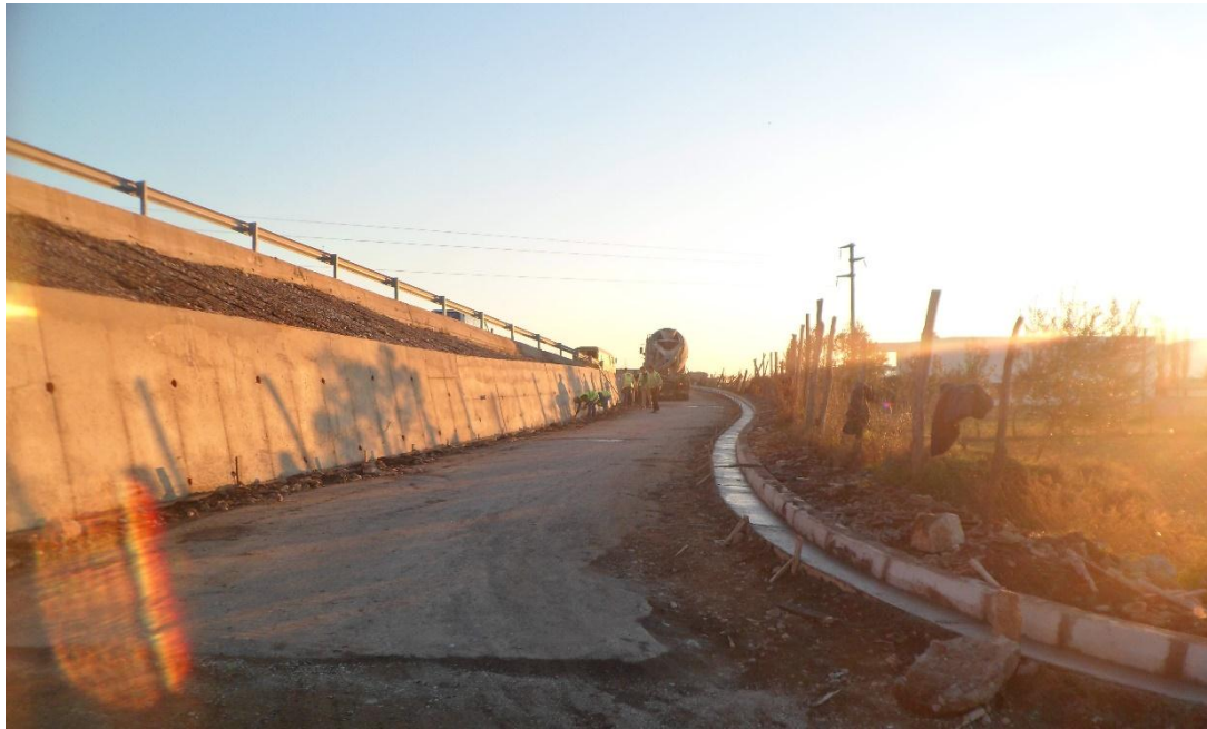
Figure 21. During work at the Overpass of the Train
