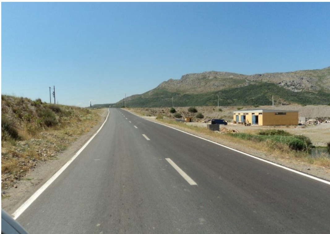
Figure 13. The Road Body of “Kiri Bridge – Mjedë” Project
