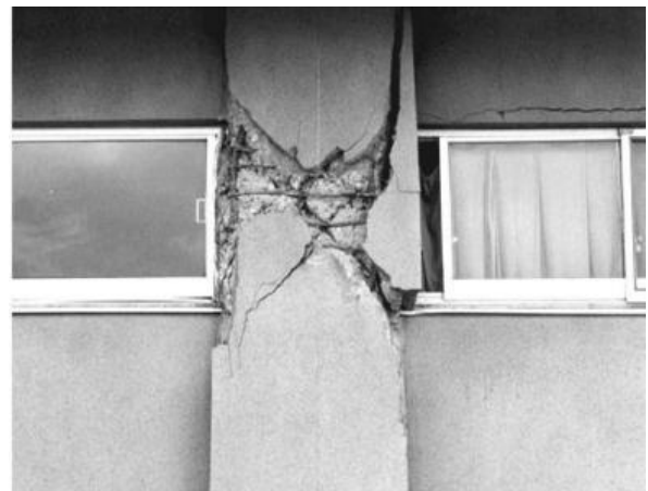
Figure 14. Short column effect created by band window [Vahidi, 2009]
