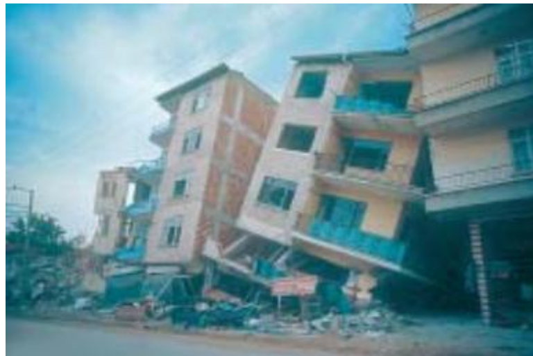
Figure 5. Sway mechanisms are often inevitable with soft story ground floors [Bachmann, 2002]
