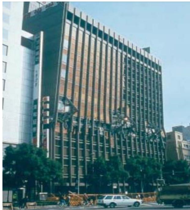
Figure 7. Failure an upper storey [Bachmann, 2002]
