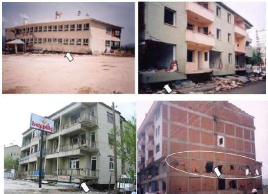
Figure 8. Building failures because of soft stories in Turkey during Bingol earthquake 2003 [Varadharajan, 2014]
