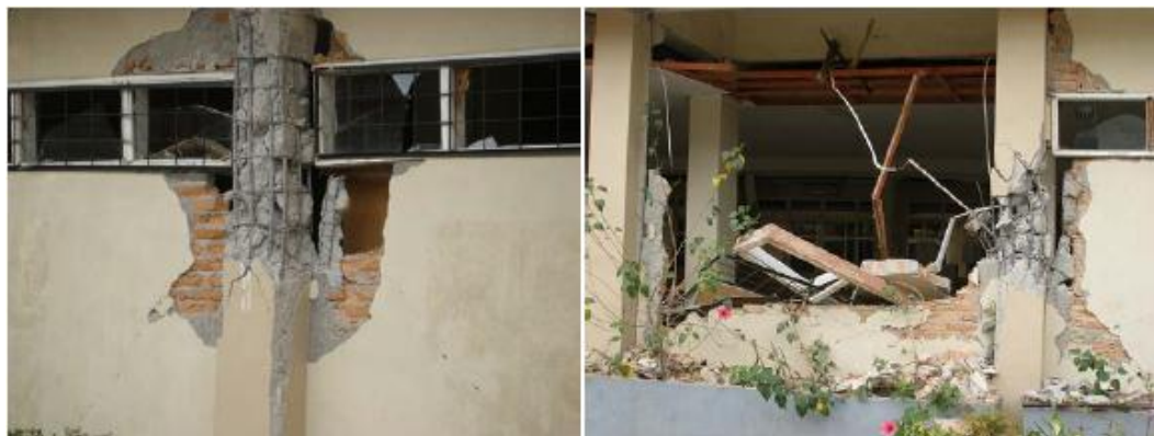
Figure 16. Building failures because of short column effect, 2009 Padang, Indonesia earthquake [Semnani, 2014]
