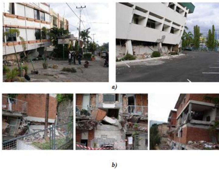
Figure 10. Soft-story collapse of infill buildings from: a) the 2009 Padang, Indonesia earthquake, b) 2009 L'Aquila, Italy earthquake [Semnani, 2014]
