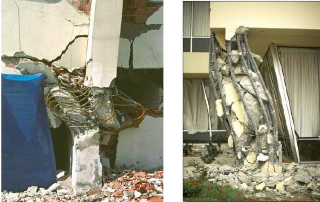
Figure 18. Failure of columns with inadequate ties, almost no confinement [Moehle et. al. , 2008]
