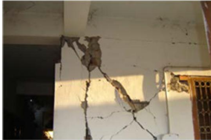
Figure 17. Building failure because of short column effect, during the 1988 Udaypur, Nepal earthquake [Semnani, 2014]
