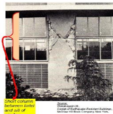
Figure 14. Short column effect created by band window [Vahidi, 2009]
