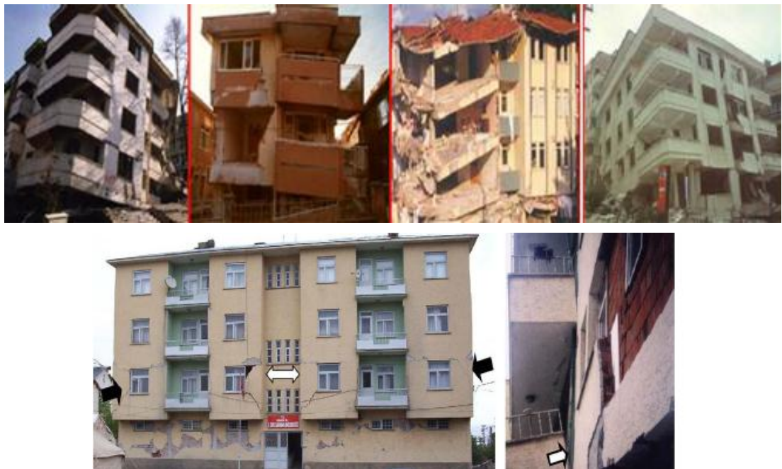
Figure 11. Failure due to overhangs [Varadharajan, 2014]
