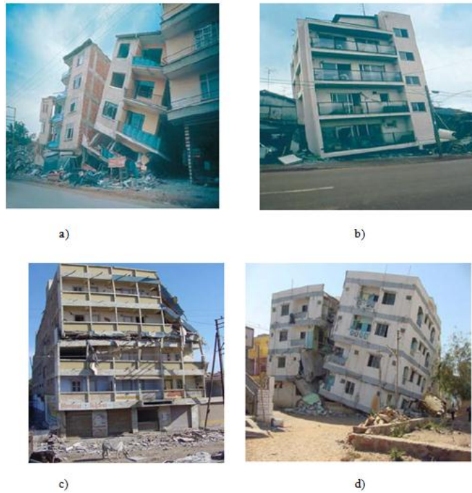
Figure 9. Building failures because of: a) Sway mechanism with soft story ground floors, b) Soft first story collapsed, c) Collapse of soft middle story, d) Vertical Split between two blocks [Semnani, 2014]
