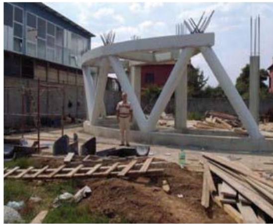
Figure 19. First Mock-Up of the building [TID archive 2016]
