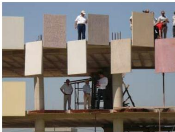
Figure 21. Second Mock-up of the building according to the project with the panel version [TID archive 2016]
