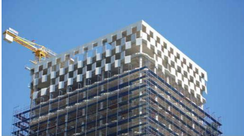
Figure 22. Mounting of panels starting from the top to the bottom, 1996 panels 600 kg each. [TID archive 2016]
