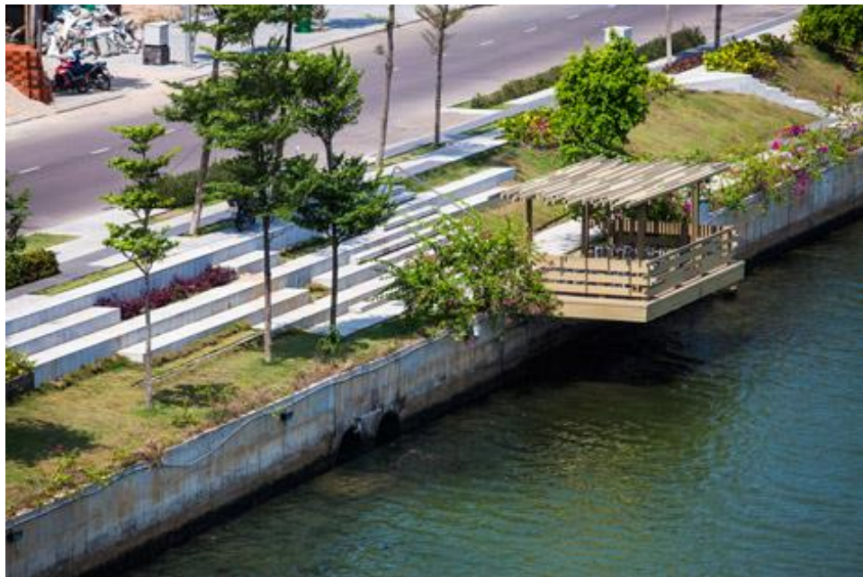
Figure 9. Wooden covered structures [Tsirintani, 2016]
