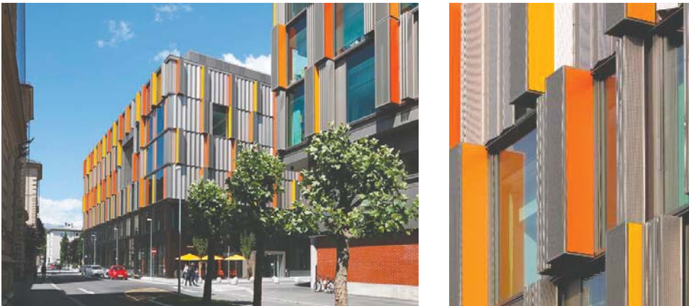
Figure 22. Pediatric and Cardiac Centre multi-layered facade panels [Nickl&Partner, 2010]
