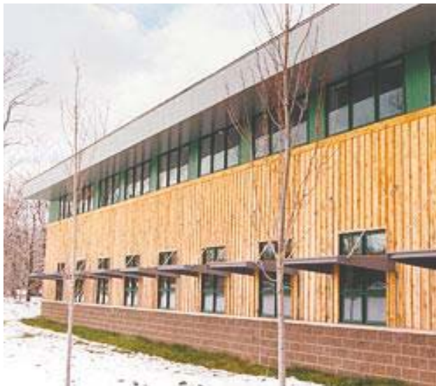
Figure 10. Cambria Office Facility exterior light shelf [Guglielmetti, Pless and Torcellini, 2010]
