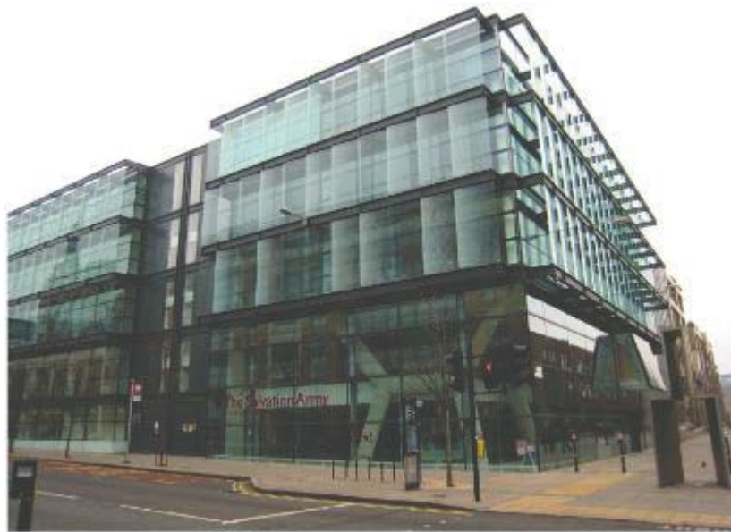
Figure 18. Laser cut panel office building, London [Public works and Government Services Canada, 2002]
