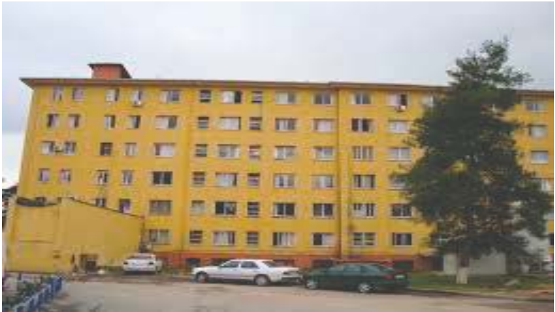
Figure 26. West Facade of Internal Diseases Hospital
