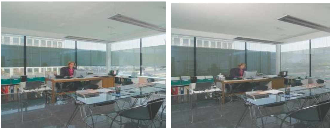
Figure 15. Sun-directing glass in the upper part of the façade. [Public works and Government Services Canada, 2002]
