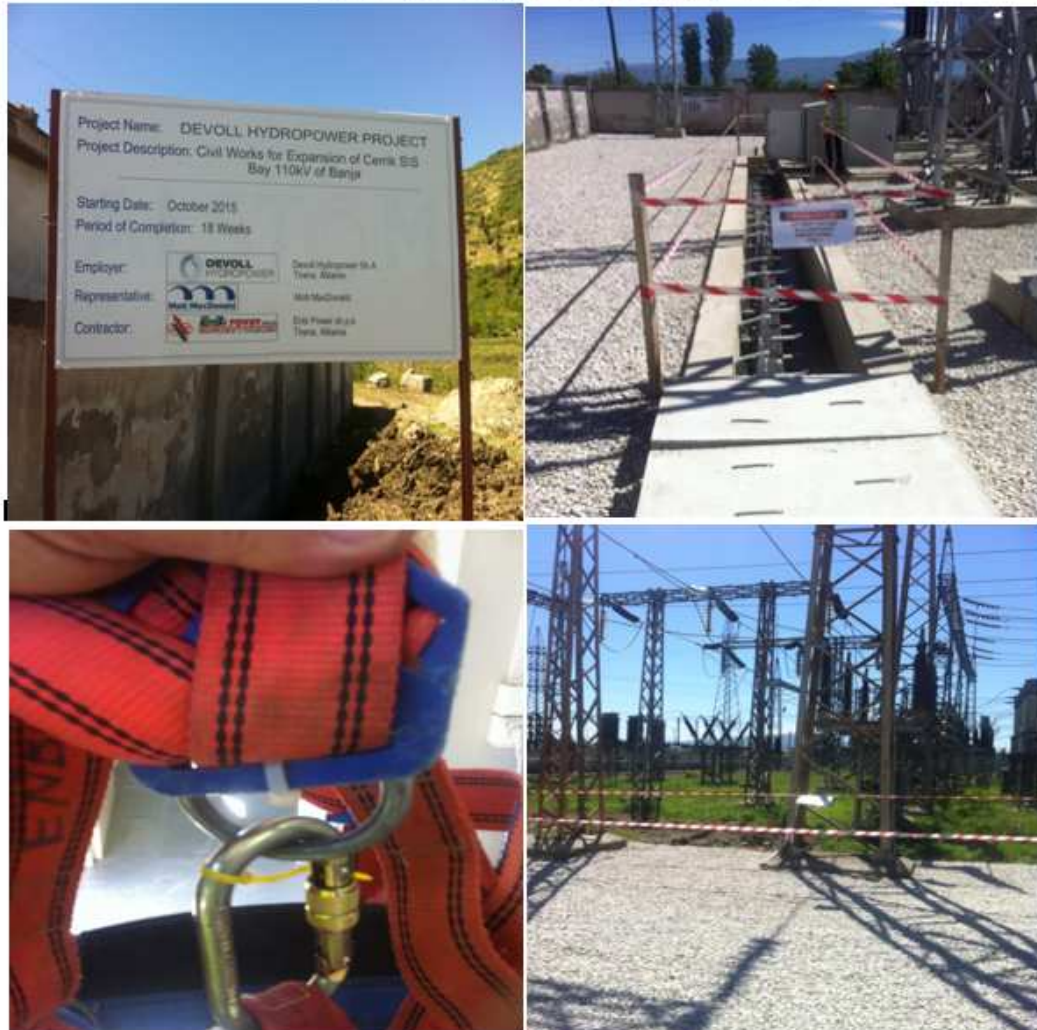
Figure 2. Corrective Measures taken for Cerrik Substation [EnBi Power].
