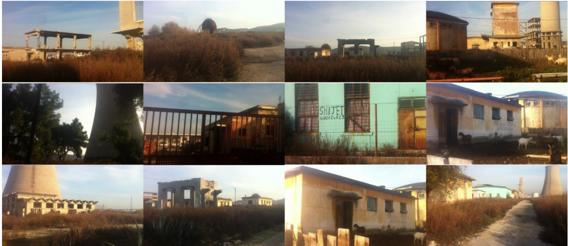
Figure 39. Site images, Ammonium Nitrate Factory [Author photos]
