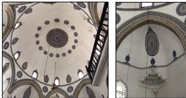
Figure 8. Interior of the dome (left) and (right) squinch on the corner [© Hadis Toçilla]
