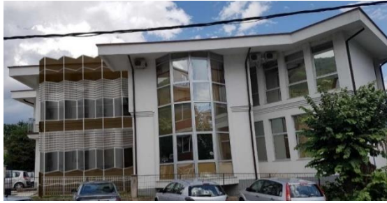
Figure 7: Appearance of the west facade of Regional and Local Administration Building located in Gostivar: provided (partly coated) double facade panels with integrated photovoltaic system B
