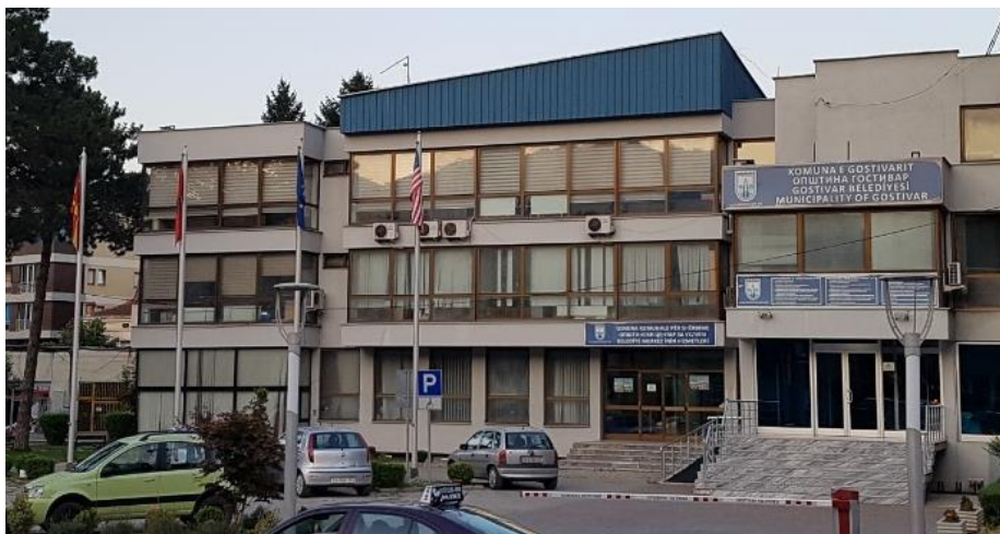
Figure 1: Regional and Local Administration Building located in Gostivar, west façade (photographed: 08.08.2017.)
