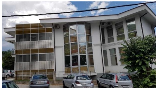
Figure 6: Appearance of the North Facade of the Regional and Local Administration Building located in Zhelino: a partially coated double facade with integrated photovoltaic panels of system A
