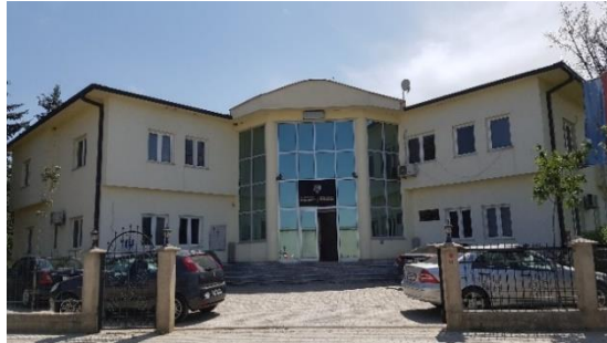
Figure 3: Regional and Local Administration Building located in Zhelino, north façade (photographed: 08.08.2017.)
