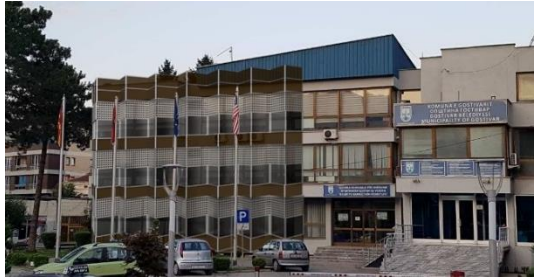
Figure 5: Appearance of the southern façade of the Regional and Local Administration Building located in Tearce: provided (partially coated) double facade with integrated photovoltaic panels of system A
