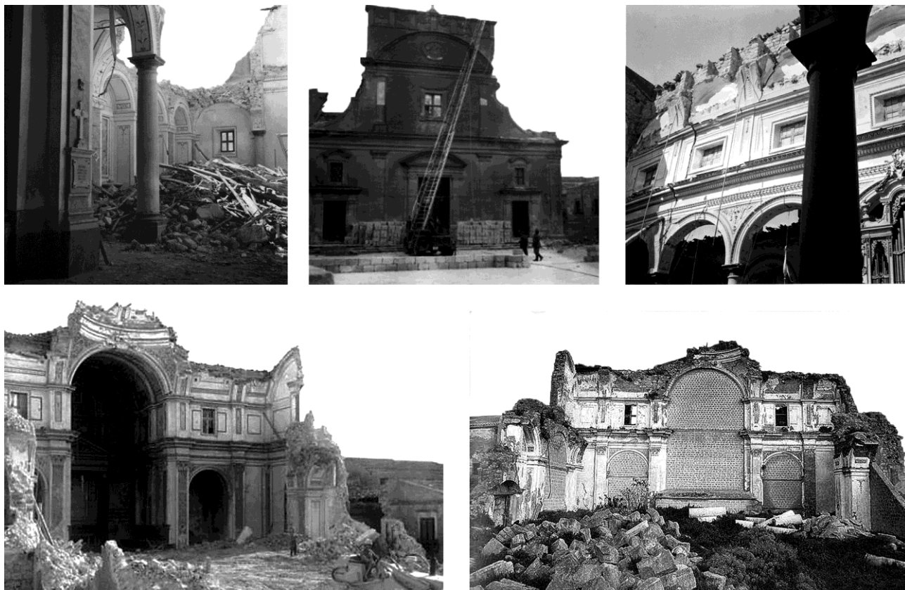
Fig. 3a: (above) The Church during demolition works. Fig. 3b: (below) The Church after demolition works.
