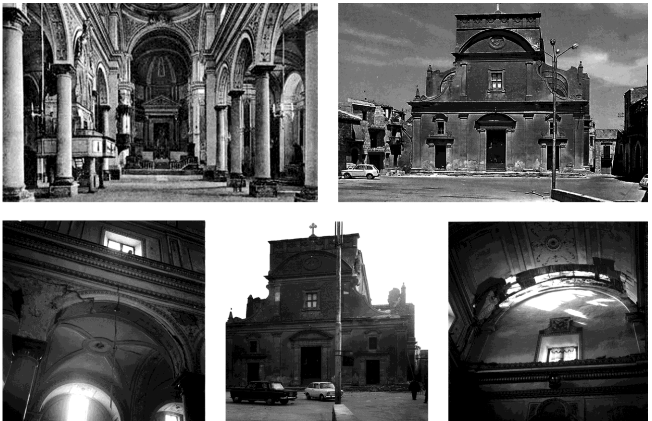
Fig. 2a: (above) The Church before the earthquake. Fig. 2b: (below) The Church after the earthquake.
