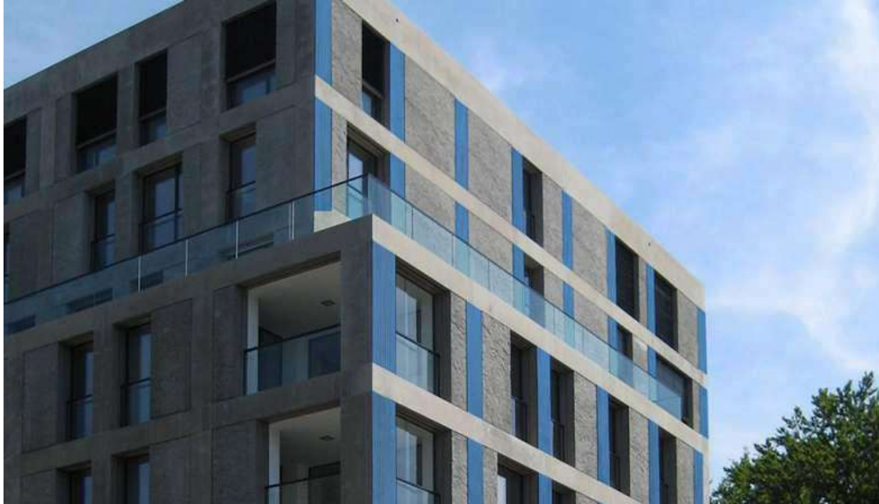
Figure 5: LafargeHolcim and Heliatek's Prefabricated Cladding with PV Film [Heliatek1].
