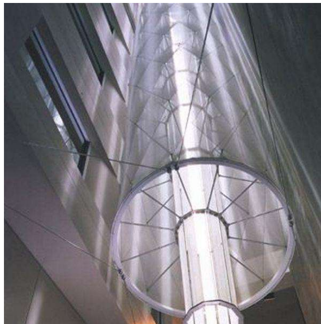
Figure 9: 36 m Solar Light Pipe in Washington DC, USA [Greendiary].
