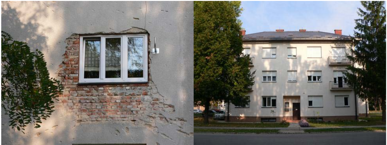
Fig. 22 (left): Visible damages on an apartment building
