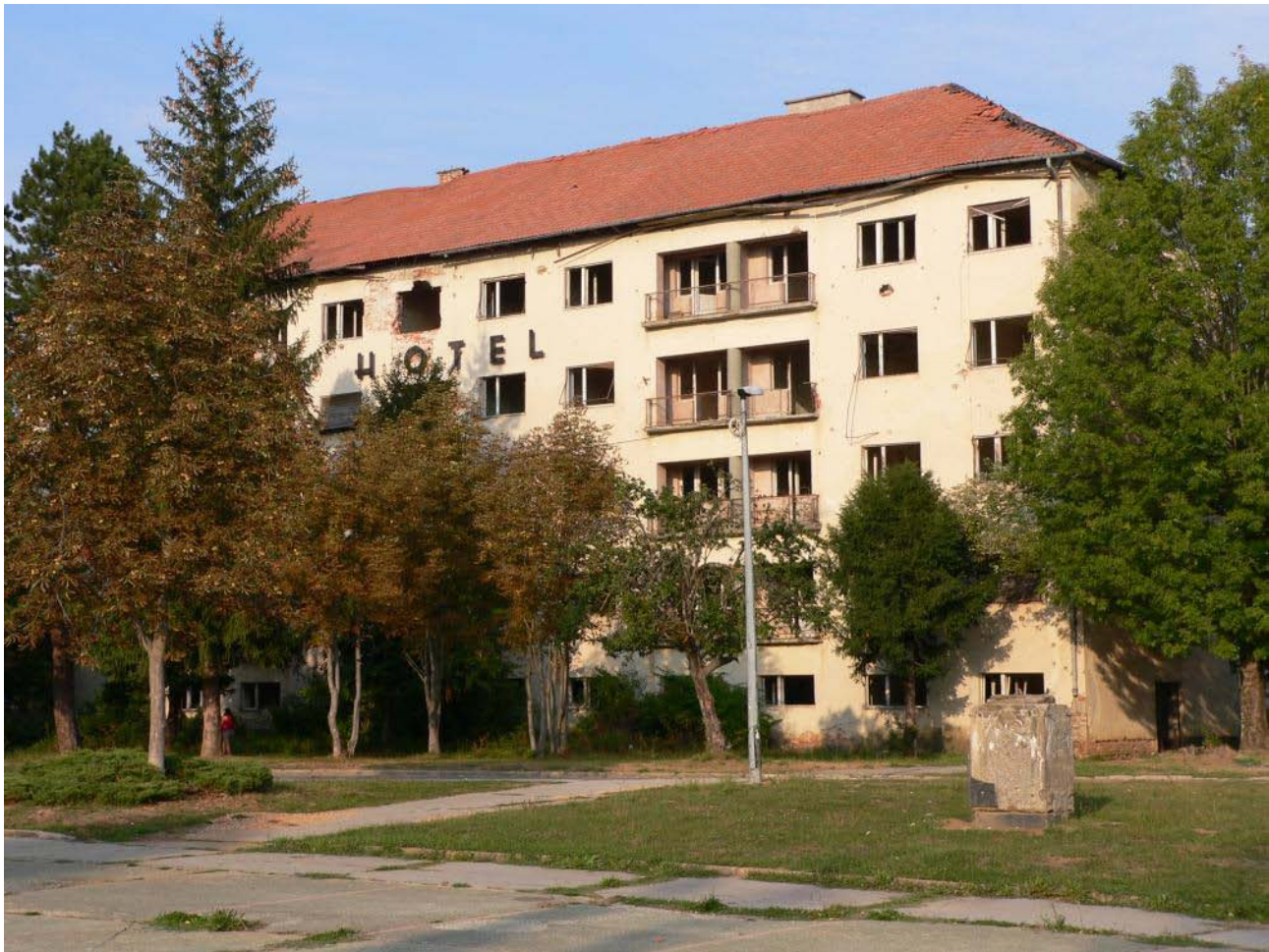
Fig. 24:Former hotel building
