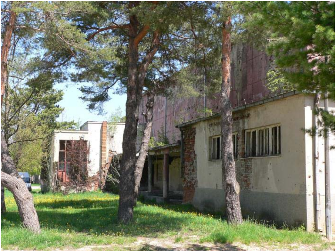
Fig. 27: Visible damages on the southern side of the Cultural Center building (2010)
