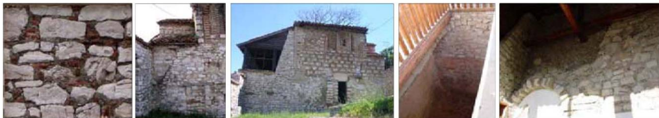
Fig. 16: 1-type of masonry of this phase, 2-traces of walled-up door in the north elevation, 3-south elevation, 4- view of cocciopesto plaster in the cistern area, 5-traces of three arches in the west elevation of the naos
