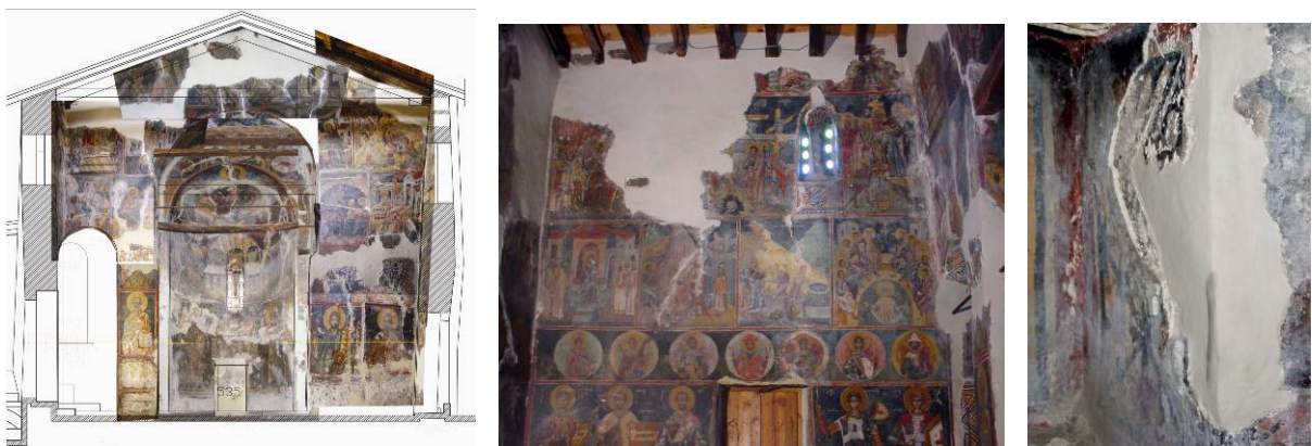
Fig. 6: Section B-B facing altar-frescoes rendered in photographic relief image (left), Frescoes in north elevation, Two layers of fresco (right)
