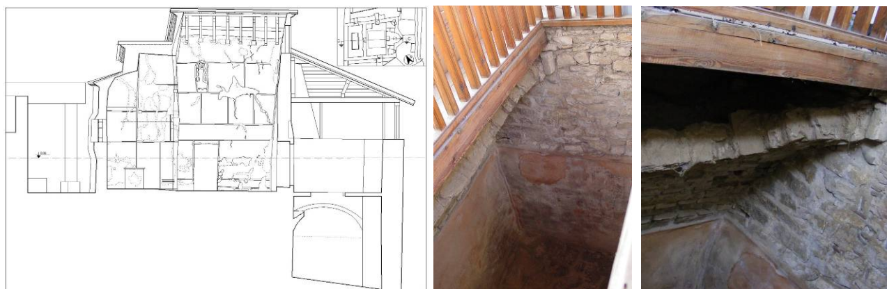
Fig. 8: Section C-C showing the location of the cistern (left) and views of the remaining structure of the cistern (right)
