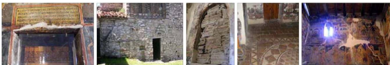
Fig. 17:1-inscription in the upper part of the door connecting the naos to the narthex, 2-traces of walled-up door in north elevation, 3-traces of walled-up entrance to the diaconicon, 4-view of pavement in stone and bricks, 5-view of the upper frame of frescoes
