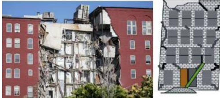
Figure 8. Collapse prevention level represents the total collapse of the structure [3]
