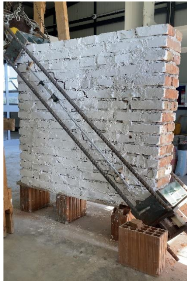
Figure 16 Failure mode of plain wall
