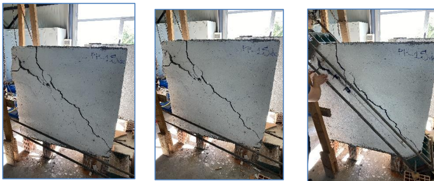
Figure 17 Failure mode of polypropylene reinforced mortar strengthened wall panel on 1 side
