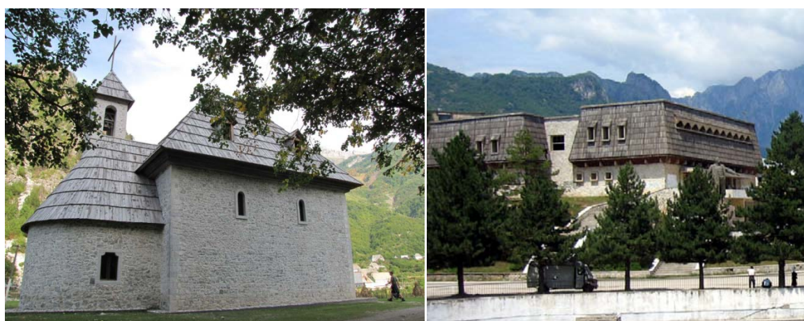
Fig 4. Building in traditional architecture of North Albania ©Donald Kokona, Barjam Curri Muzeum, ©Wikipedia
