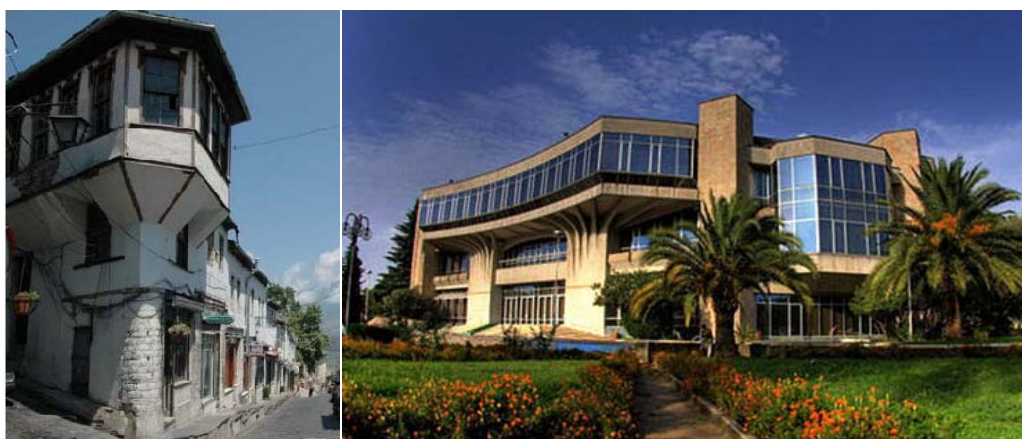
Fig3. Traditional timber frame house in Gjirokastrë served as inspiration to The Congress Palace in Tirana © Wikipedia, Nikelina Bineri
