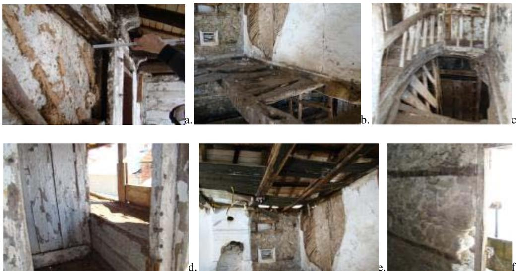
Fig. 3: a. Damaged internal wall constructed by clay reinforced with timber willows; b, c. & e. deterioration of a timber elements at ceiling/flooring and staircase structure; d. poor maintenance of planking envelope; f. misapplied of structural conservation.
