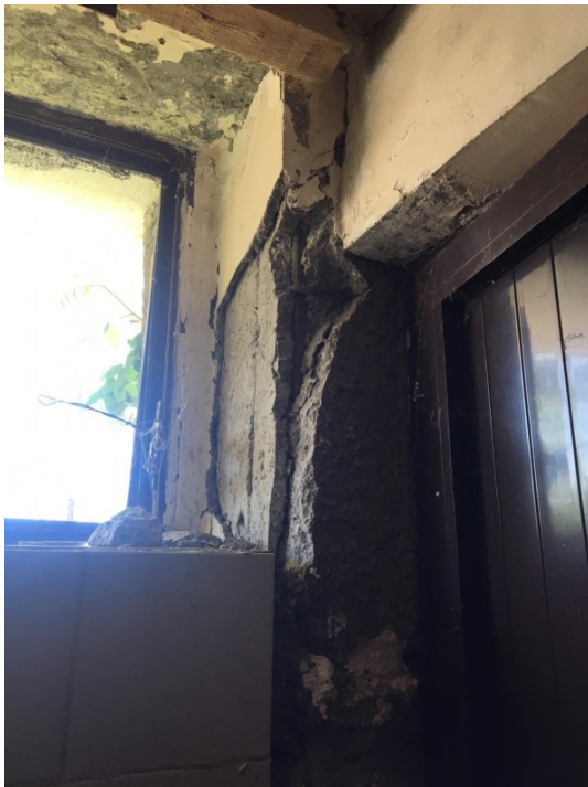
Figure 26 Column Damage
