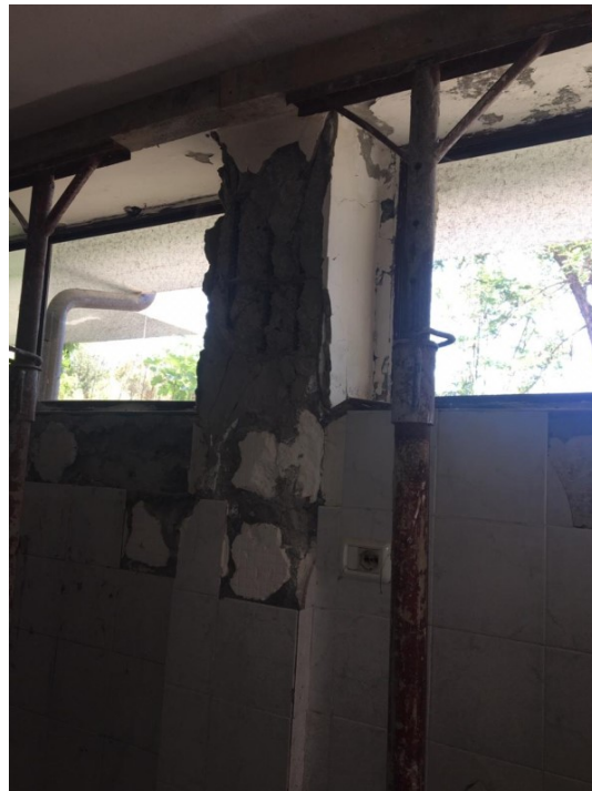
Figure 24 Column Damage
