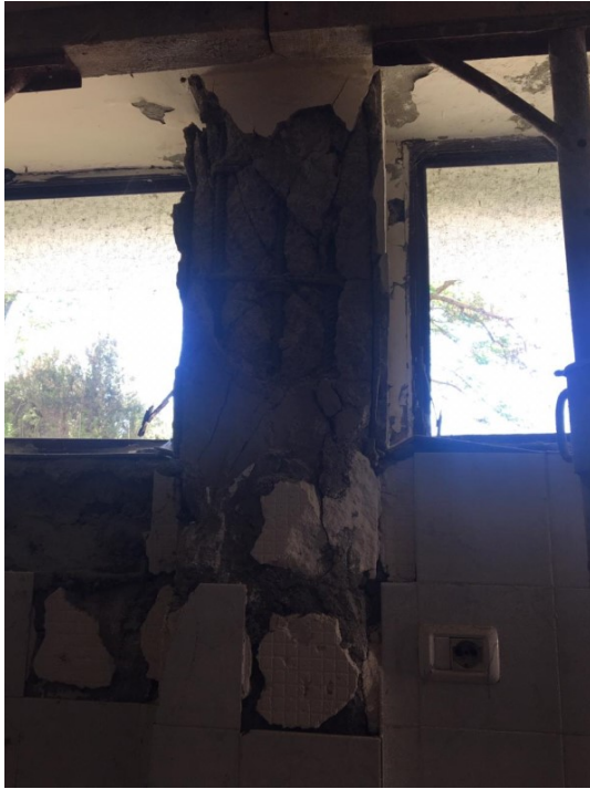
Figure 25 Column Damage
