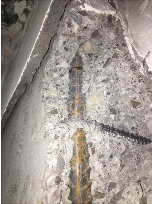
Figure 27 Reinforcement Uncover
