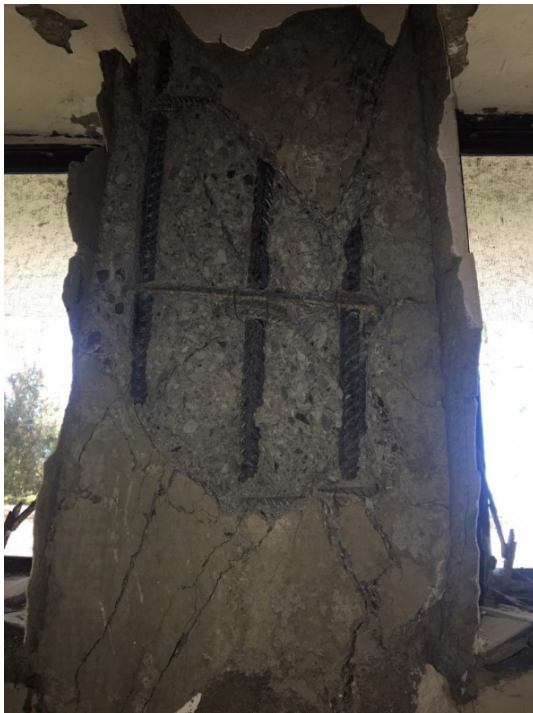
Figure 28 Reinforcement Uncover
