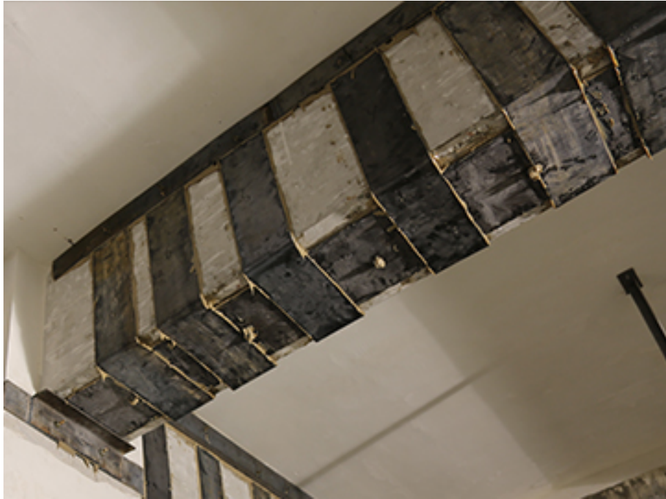
Figure 13 Steel Plate Strengthening of Beams
