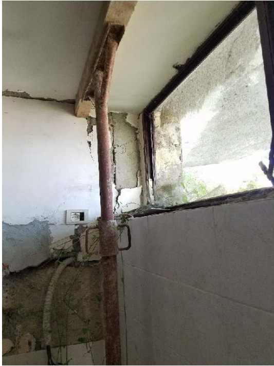
Figure 31 Column Damage
