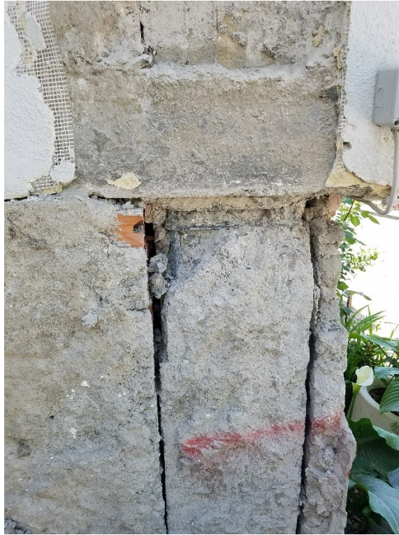
Figure 33 Column Damage
