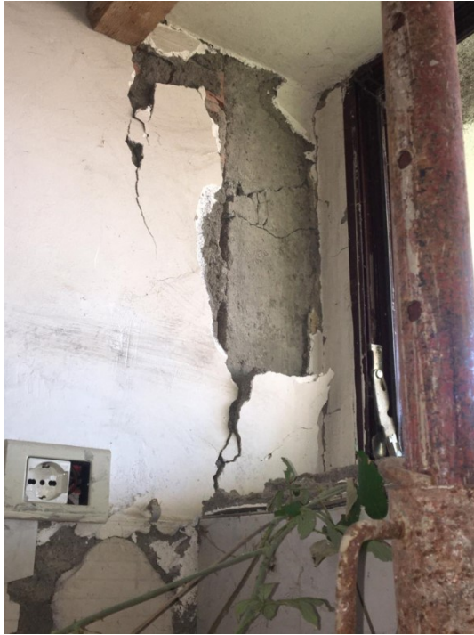
Figure 29 Column Damage
