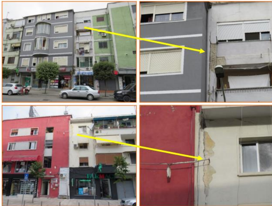
Figure 5 Pounding failure due to lack of dilatation joints (Bilgin, Leti, Hysenlliu, & Bidaj, 2020)
