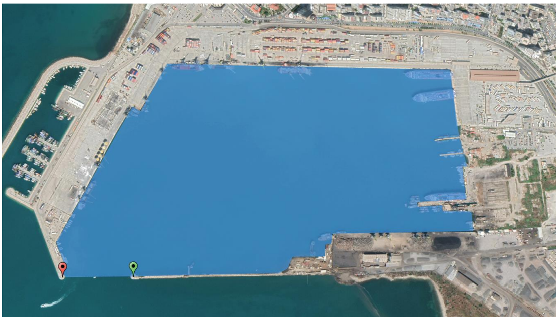
Figure 6 - Port basin and the red and green lights that delimit the port entrance
