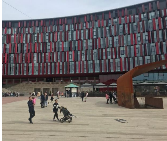
Figure 21. The ticket stand, the café's outdoor and the stairs' canopy. Courtesy of the author
