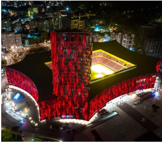
Figure 118. Air Albania Stadium in Tirana, Albania.
