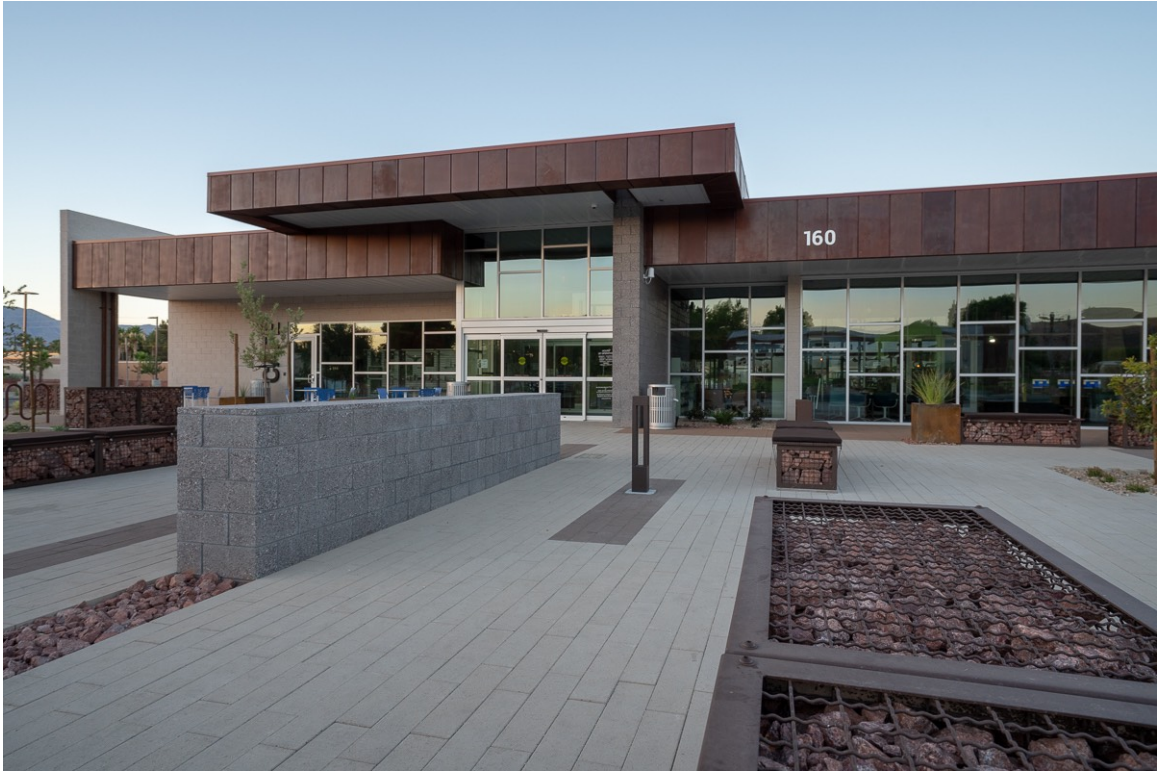
Figure 30- Photo of the facade
