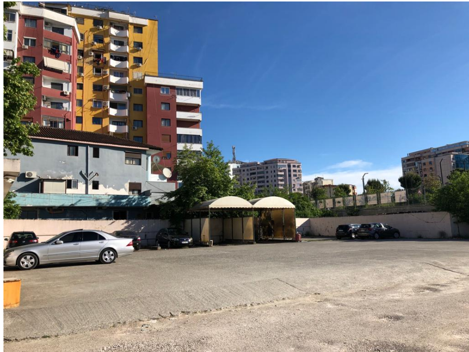
Figure 46- Photos of the site
