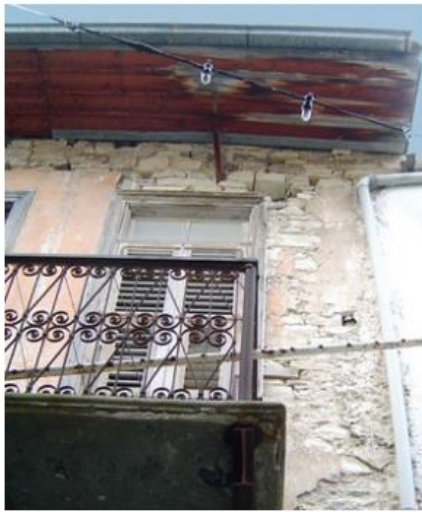
Situation before works
