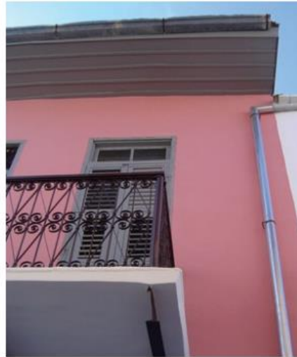
Situation after works
