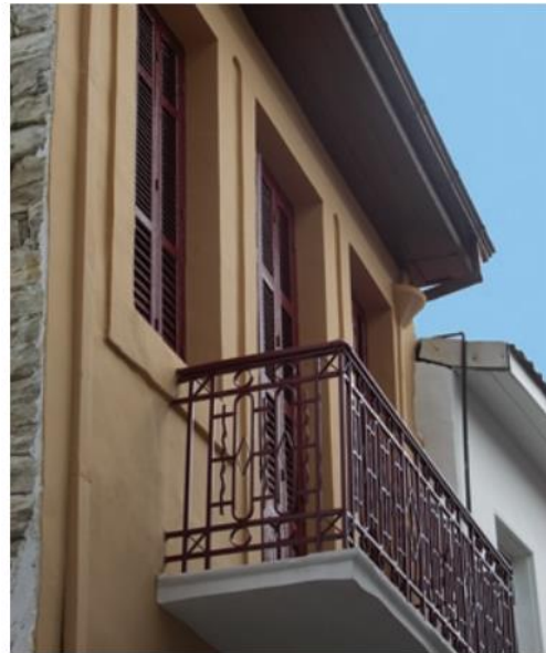
Situation after works
