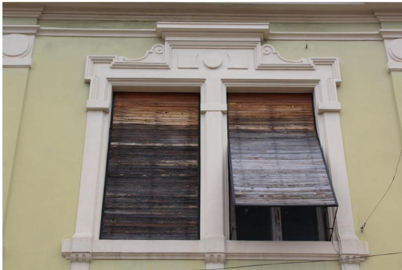
Figure 23 degradation of shutters, courtesy of the author, 2021
