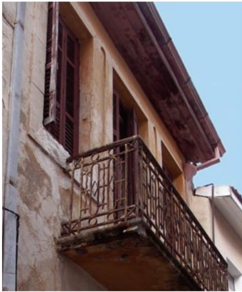
Situation before works
