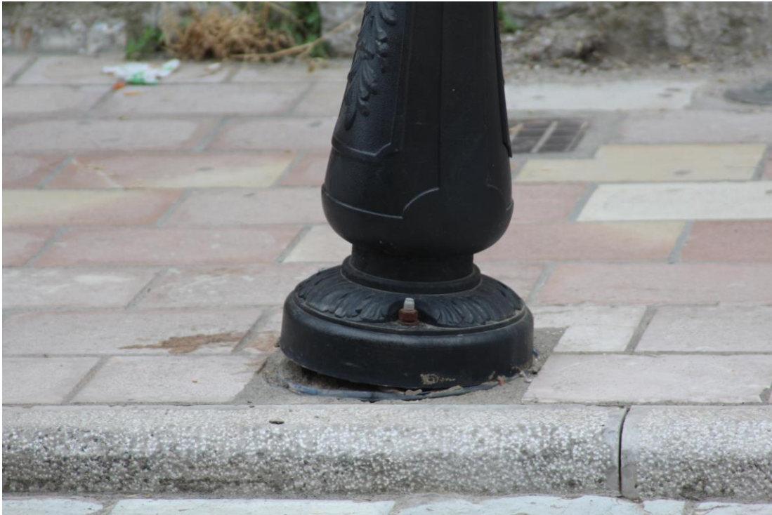
Figure 24 current condition of road lighting, courtesy of the author, 2021
