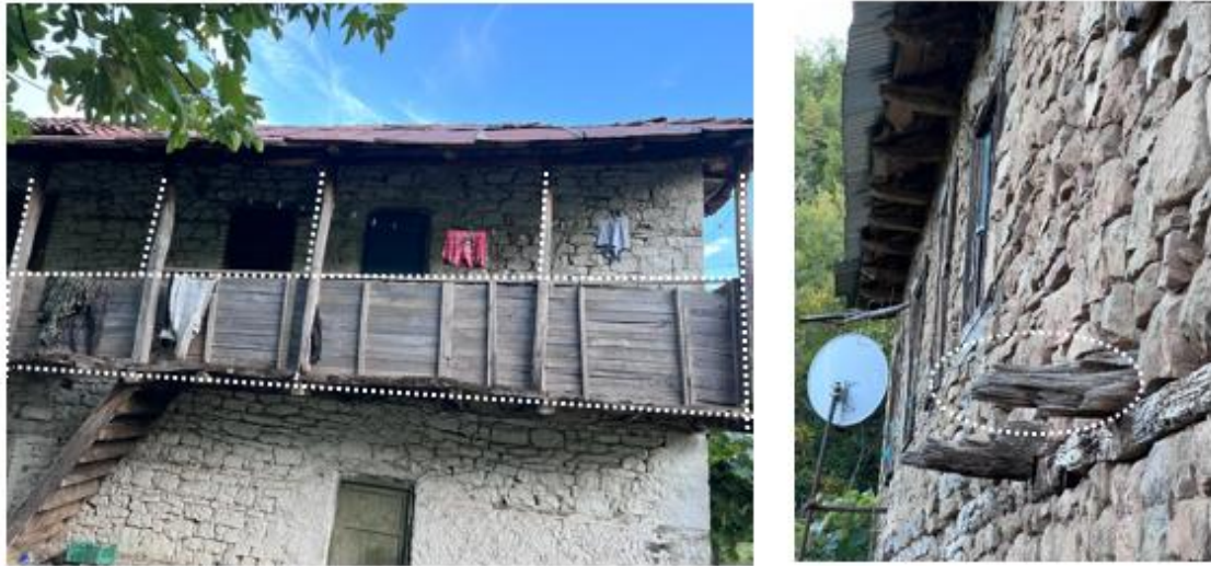
Figure 38. Existing house with “qestekë” in Shëngjin village owned by Sh.Sala and the remaining extensions of beams of what used to be a “qestekë” in a house in Shëngjin village owned by Sh.Kaloshi.
