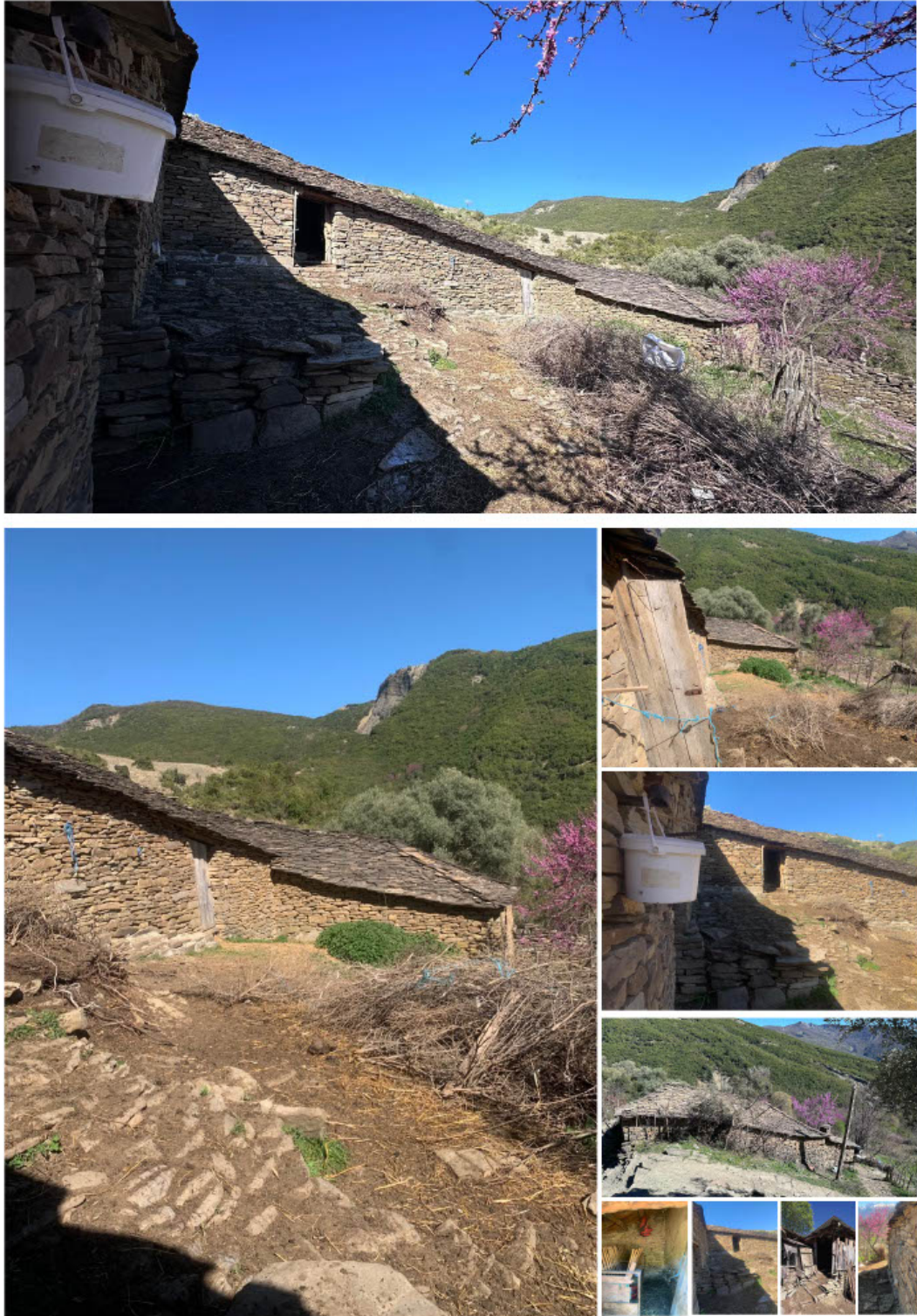
Figure 96. On-site photography of the Barn House
