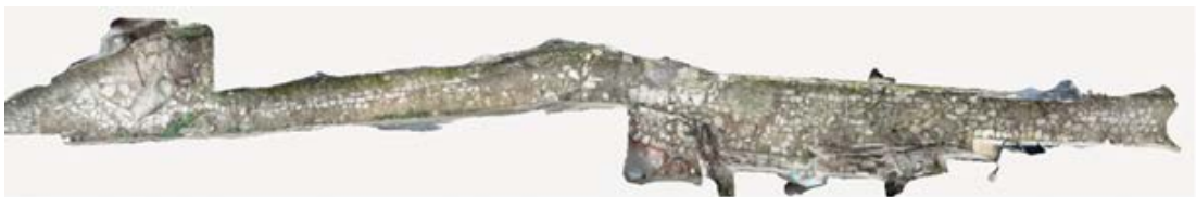
Figure 51. A 3D view of a section of road where the cobblestone pavement partly damaged
