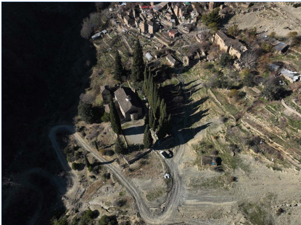
Figure 30. Aerial image of the village's main entrance
