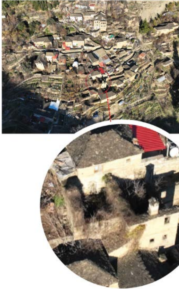
Figure 110. Identification of the existing conditions
