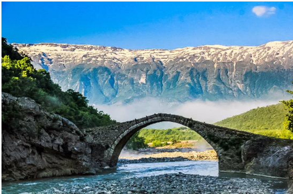
Figure 36. Katiu Bridge, surrounded by natural thermal springs
