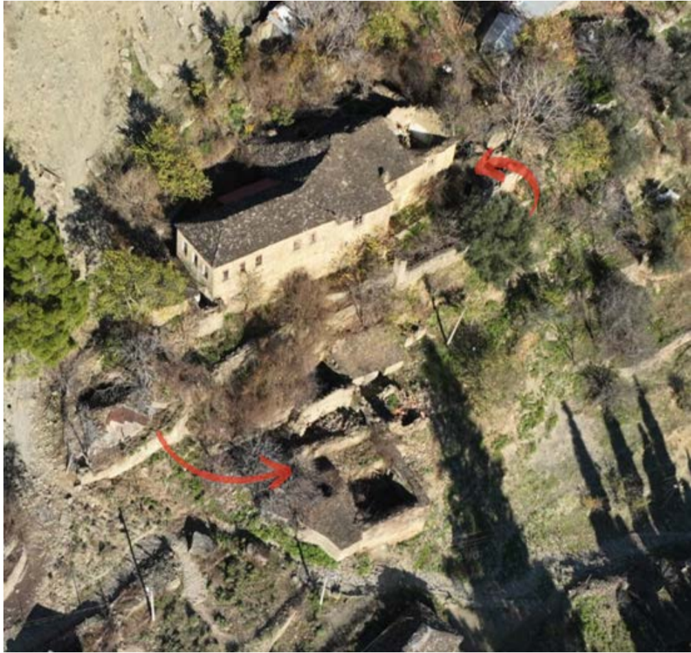
Figure 101. Ruins of burnt house
