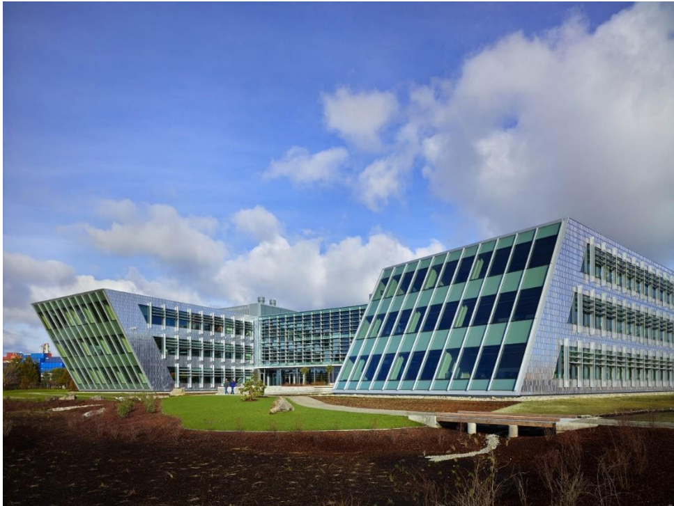
Figure 13: Federal Center South Building 1202 [15]
