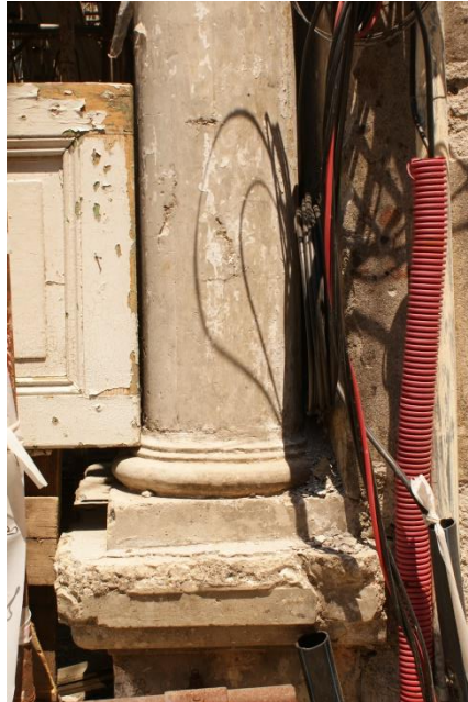
Fig. 1. 1 Detail of façade column of “Kafja e Madhe” (author)
