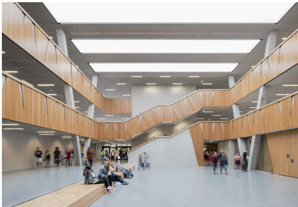
Figure 5: Velux Modular “Longlights” resining on top of the atrium, used for ventilation and daylight
