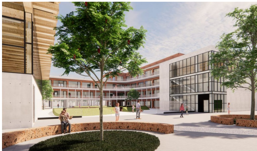
Figure 24: The outer façade of the school with external shading devices
