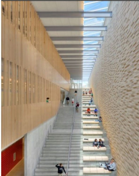
Figure 15: The three stores atrium for ventilation and natural daylight
