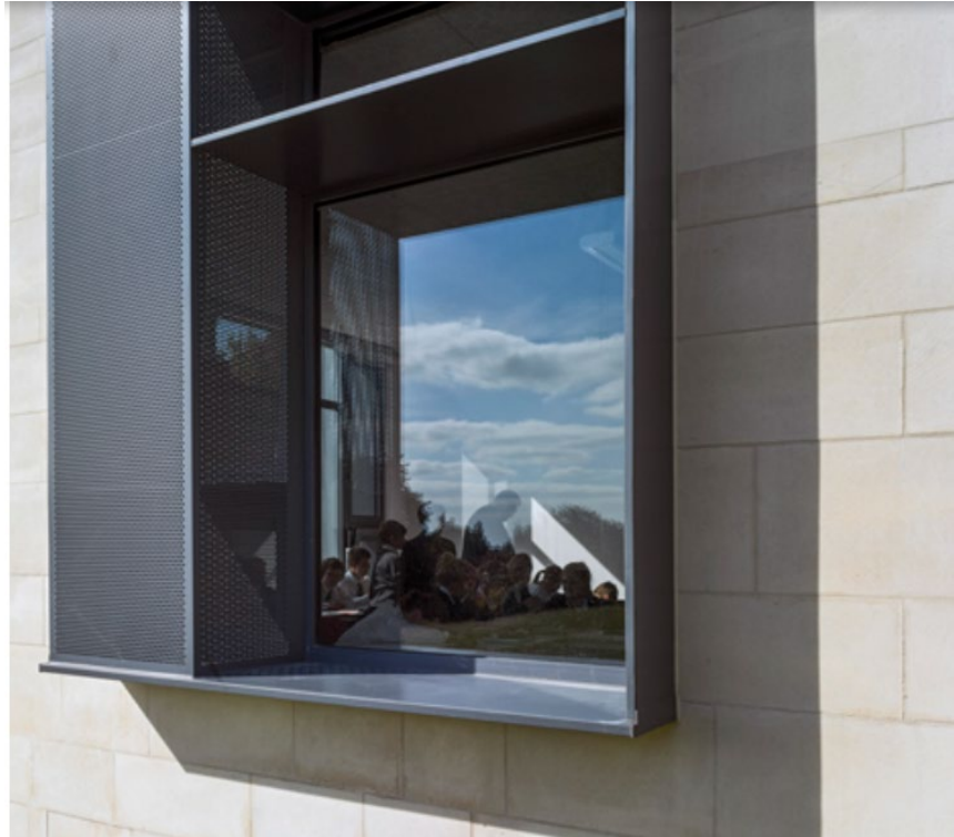
Figure 12: The windows surrounded by grey frames and perforated panels
