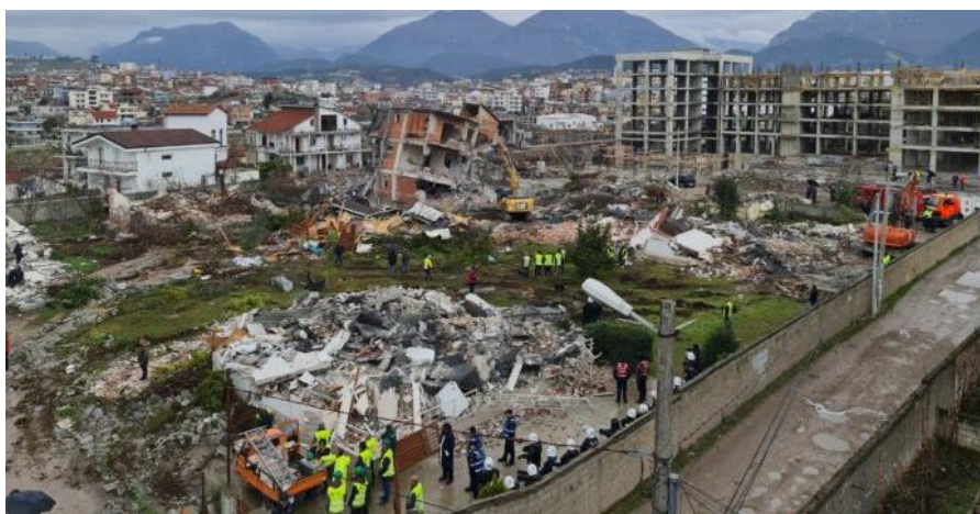
Figure 31: Demolition of buildings in "5Maji".
