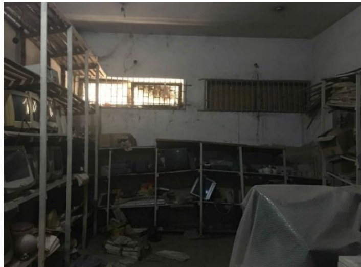
Figure 5. 5/a/b. Pictures from the basement.
