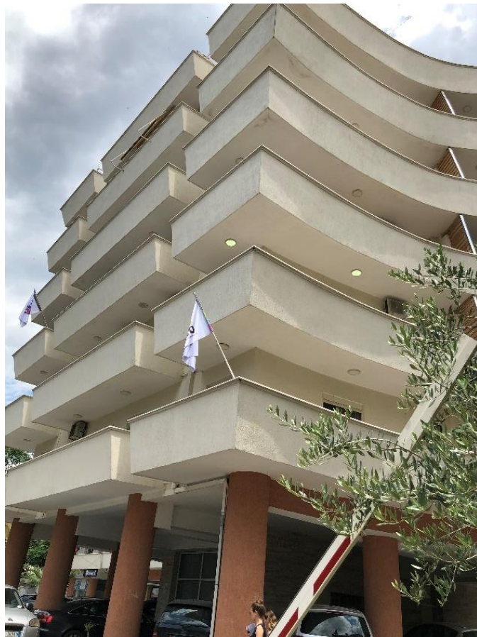
Figure 281. Balcony typology on the site (33)
