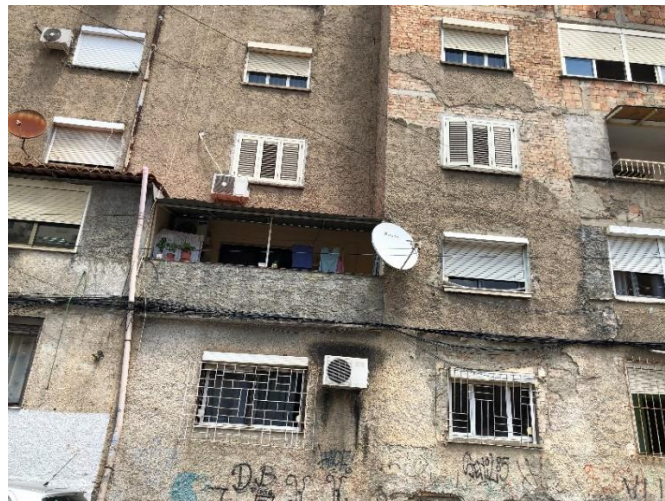
Figure 220. Balcony typology on the site (25)
