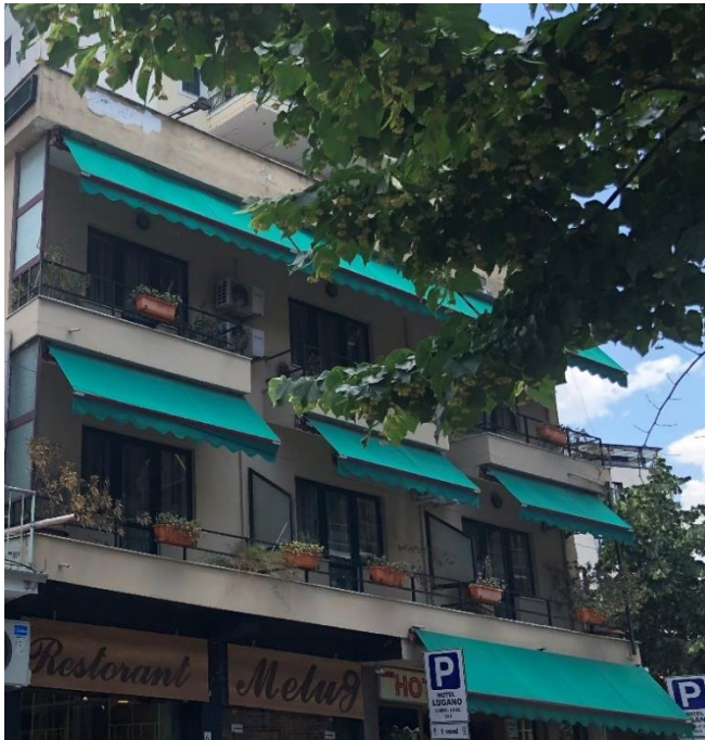
Figure 262. Balcony typology on the site (12)
