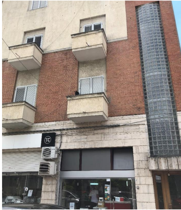
Figure 272. Balcony typology on the site (22)
