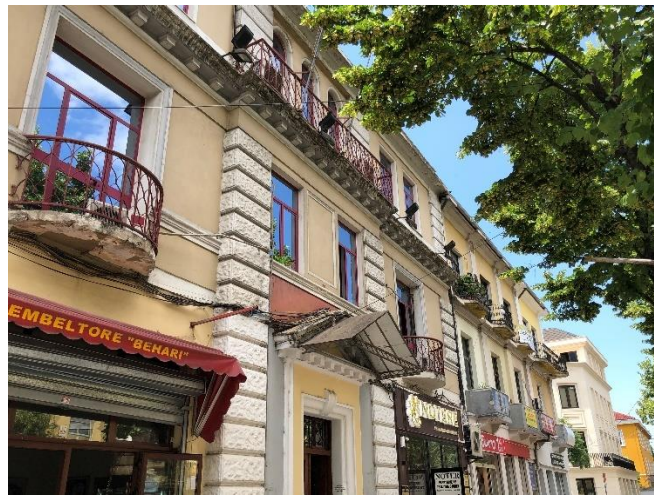
Figure 219. Balcony typology on the site (11)
