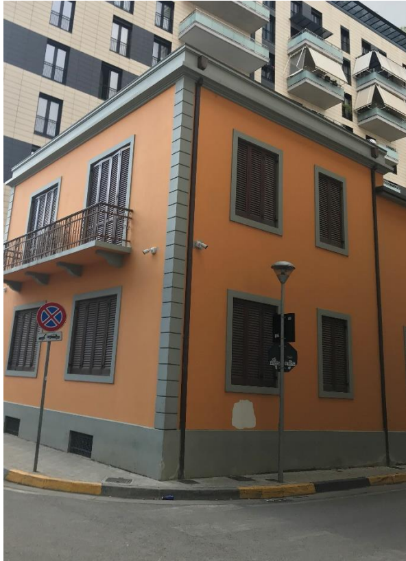
Figure 171. Street edge element in “Kajo Karafili” street
