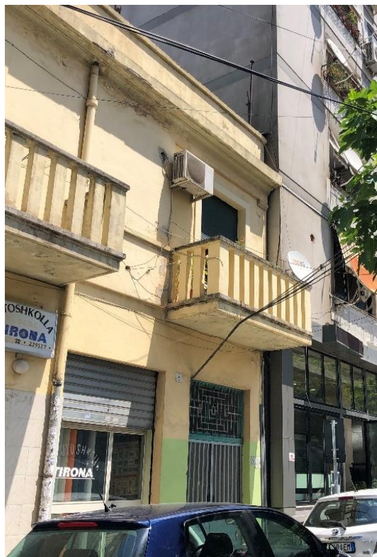
Figure 256. Balcony typology on the site (5)
