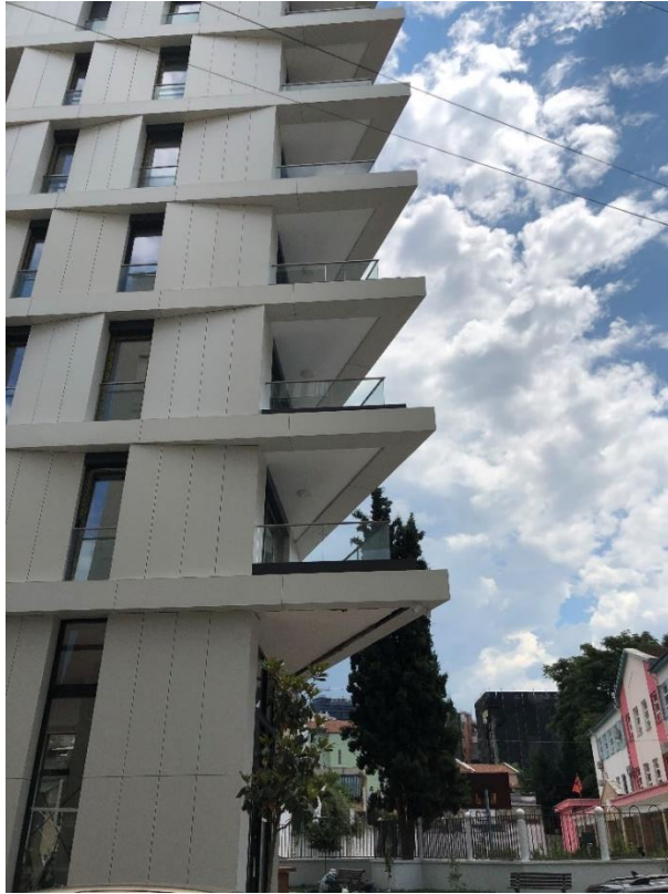
Figure 221. Balcony typology on the site (27)
