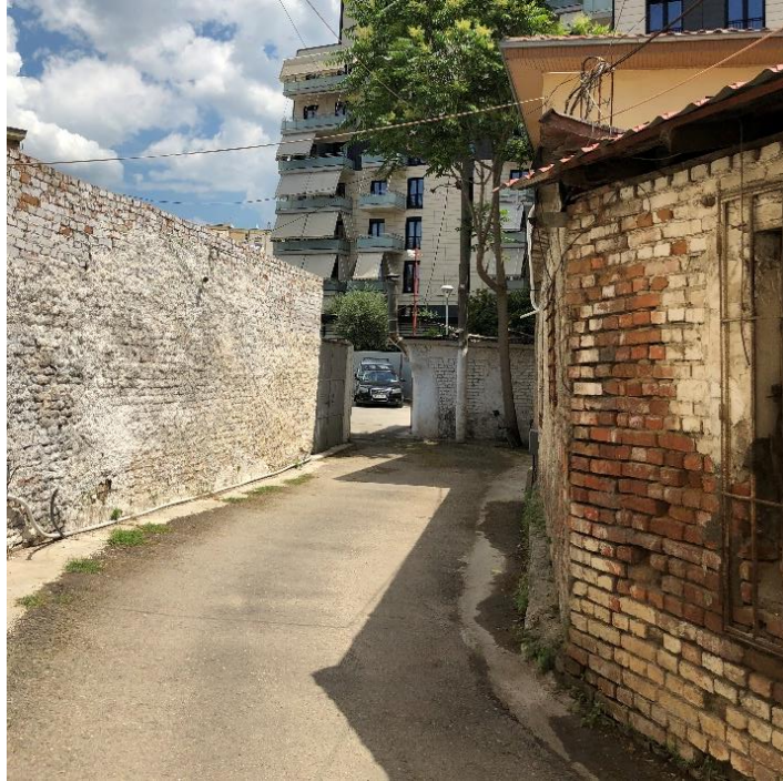
Figure 242. Front entry surrounded by walls (9)
