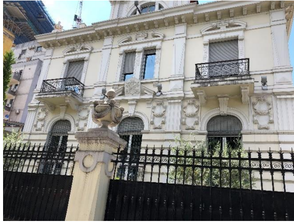
Figure 259. Balcony typology on the site (8)
