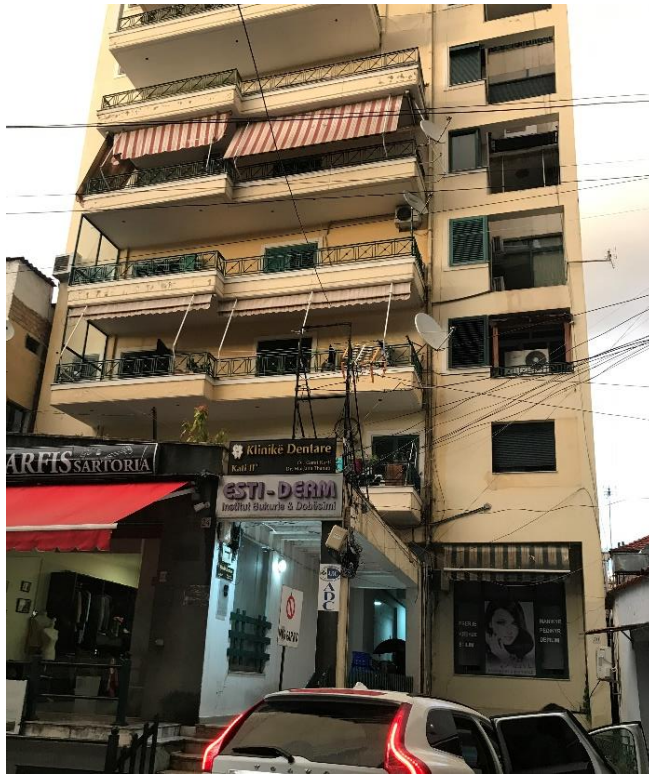
Figure 263. Balcony typology on the site (13)
