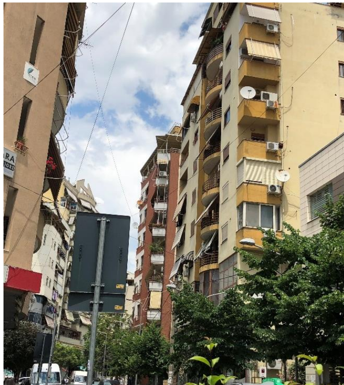
Figure 277. Balcony typology on the site (29)
