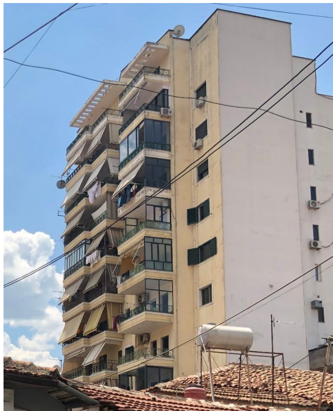
Figure 271. Balcony typology on the site (21)
