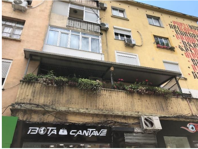
Figure 261. Balcony typology on the site (10)
