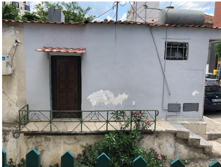
Figure 226. Terrace on the street (4)
