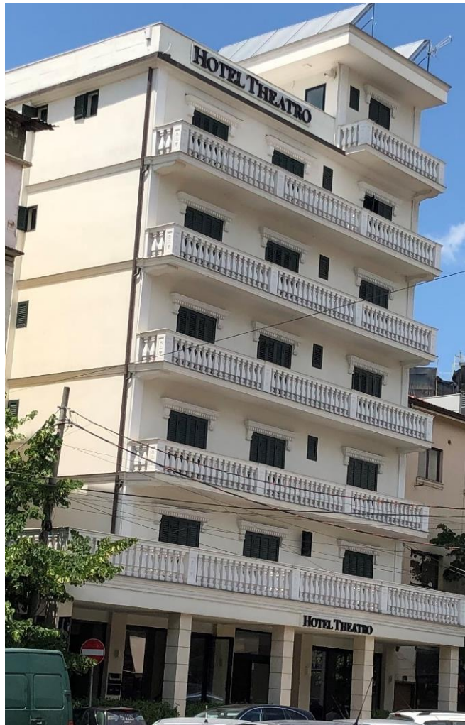
Figure 265. Balcony typology on the site (15)
