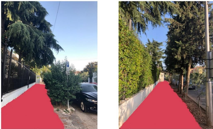
Figure 158. Sidewalk typology in "Skanderbeg" street
