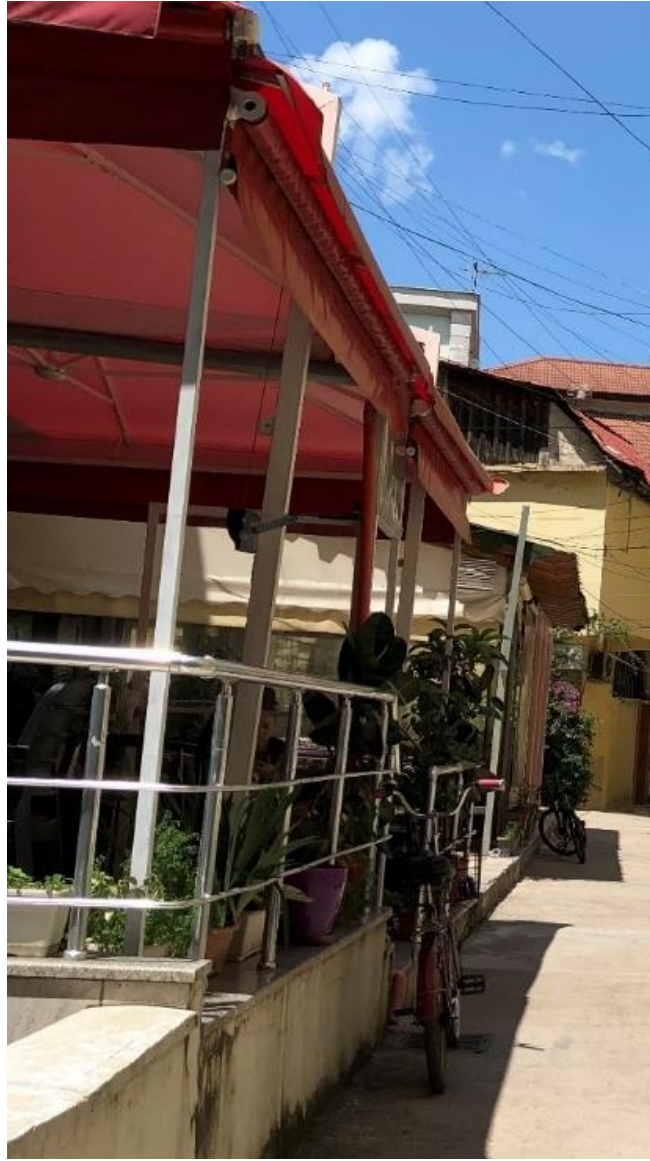
Figure 223. Terrace on the street (1)
