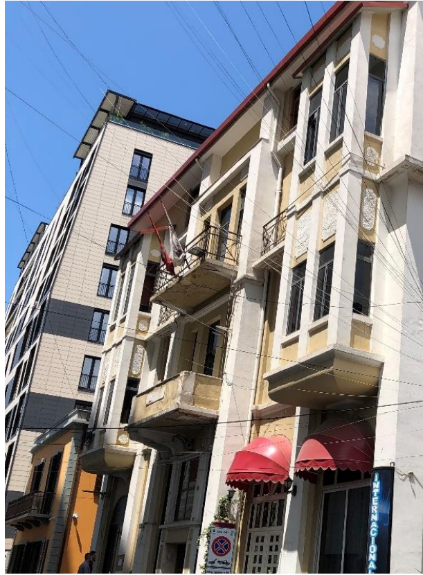
Figure 257. Balcony typology on the site (6)
