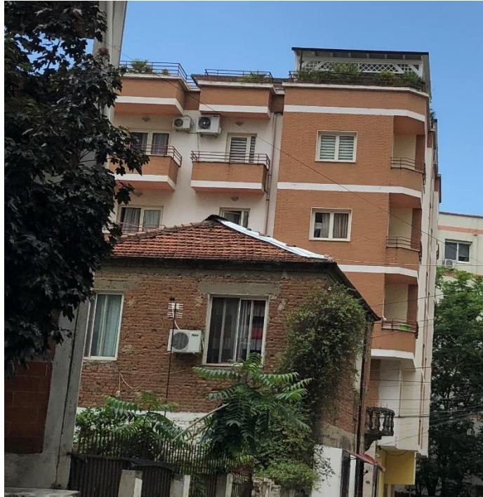
Figure 280. Balcony typology on the site (32)
