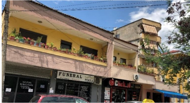
Figure 267. Balcony typology on the site (17)
