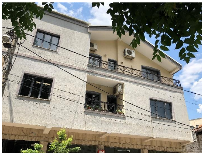
Figure 266. Balcony typology on the site (16)
