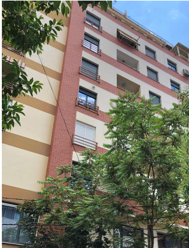
Figure 276. Balcony typology on the site (28)
