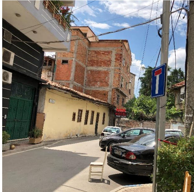
Figure 297. Front entry surrounded by walls (23)
