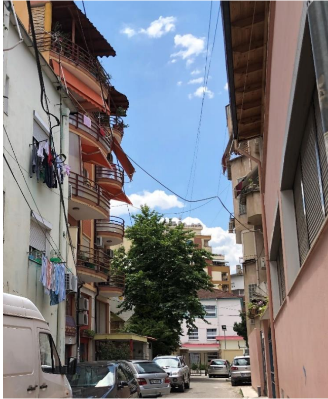
Figure 274. Balcony typology on the site (24)
