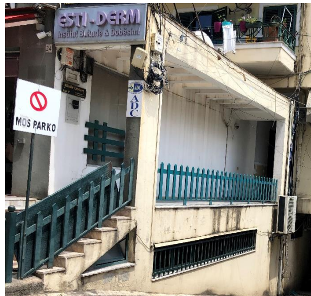
Figure 287. Raised entry and entrance hall (11)
