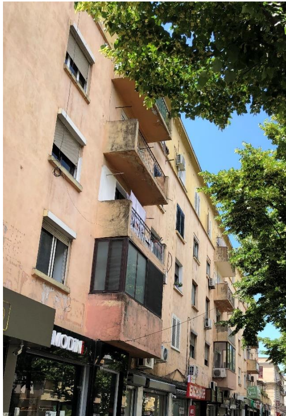
Figure 260. Balcony typology on the site (9)
