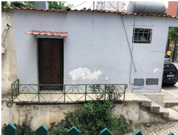
Figure 243. Raised entry and entrance hall (10)
