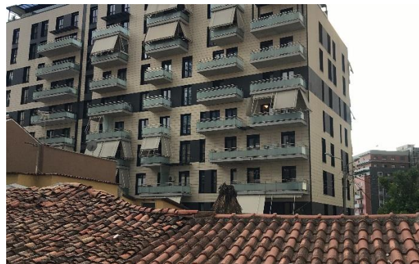
Figure 258. Balcony typology on the site (7)
