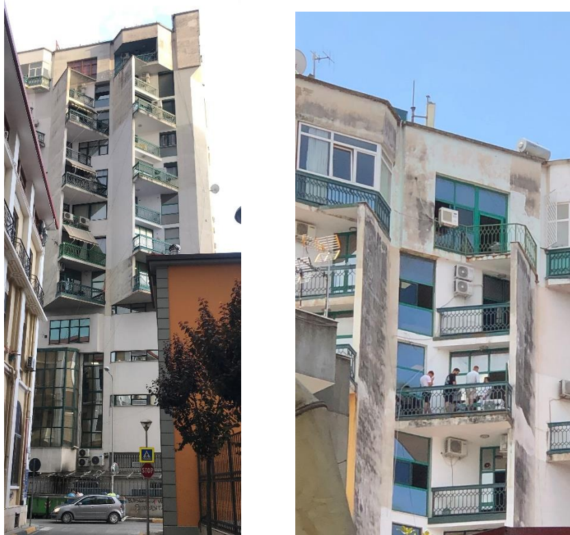
Figure 255. Balcony typology on the site (4)
