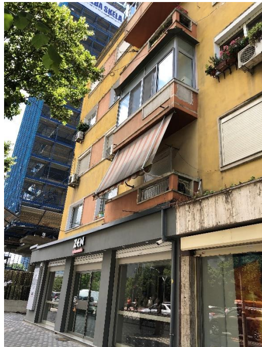
Figure 212. Balcony typology on the site (1)
