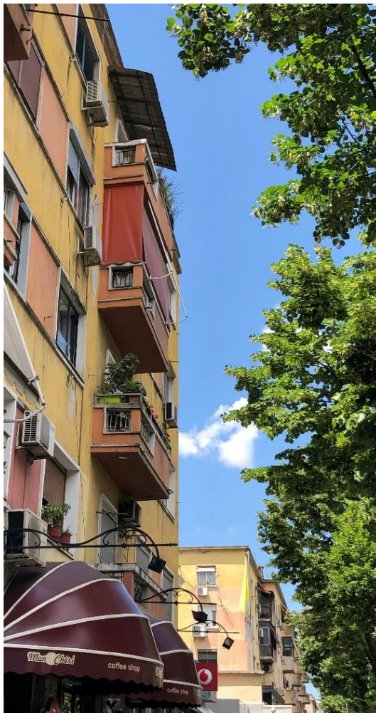
Figure 254. Balcony typology on the site (3)
