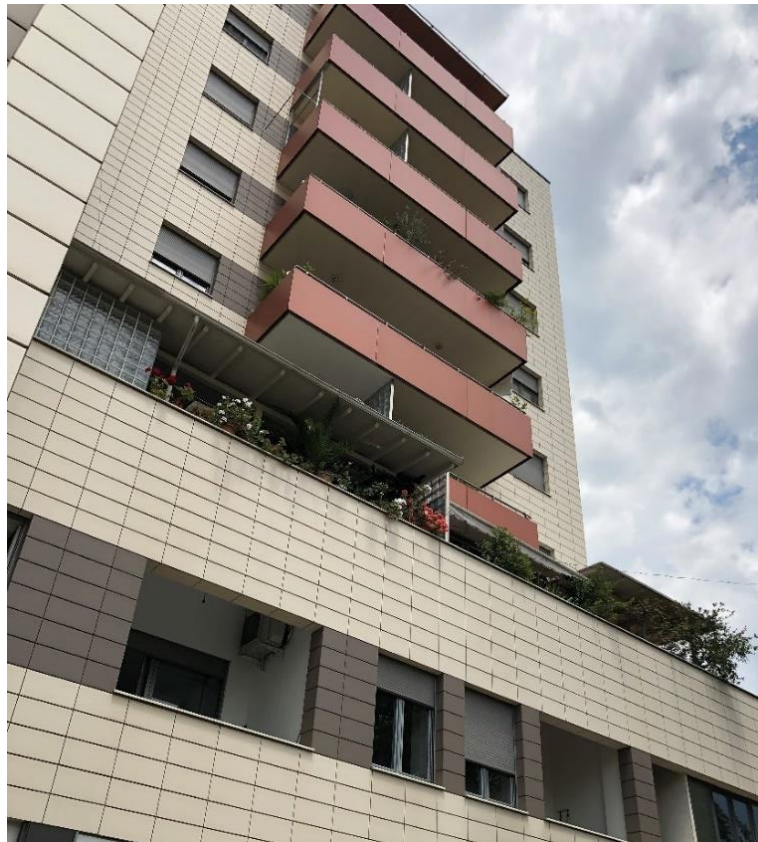
Figure 279. Balcony typology on the site (31)
