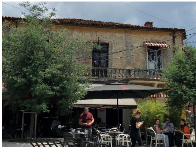
Figure 268. Balcony typology on the site (18)
