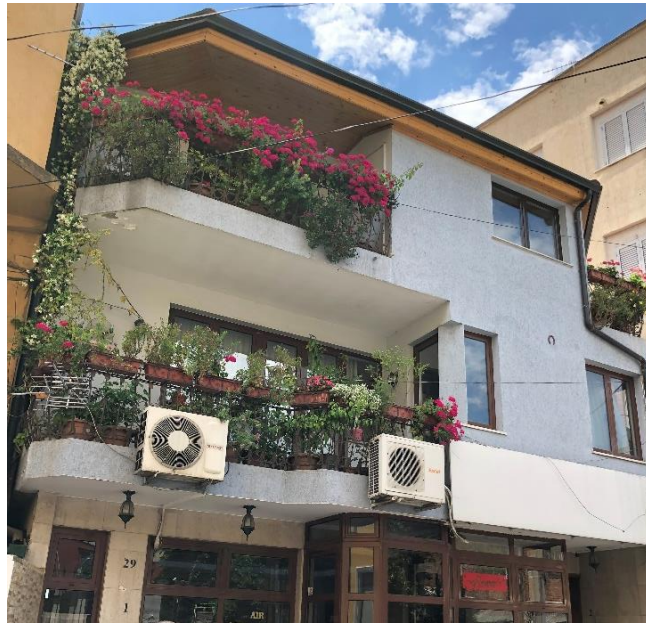
Figure 270. Balcony typology on the site (20)
