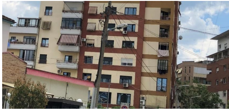
Figure 278. Balcony typology on the site (30)
