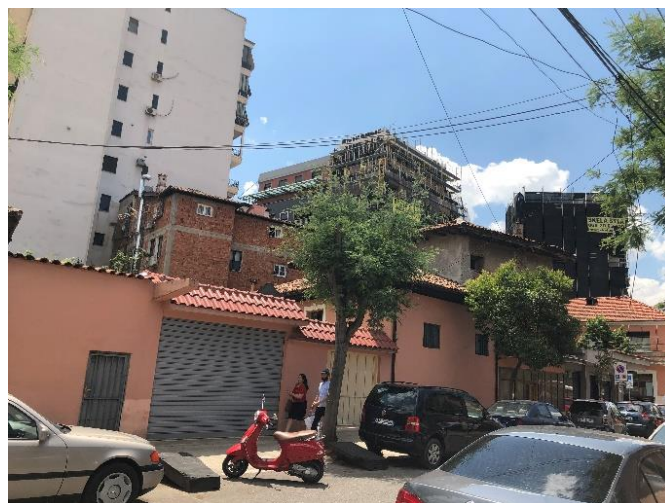
Figure 288. Front entry surrounded by walls (12)
