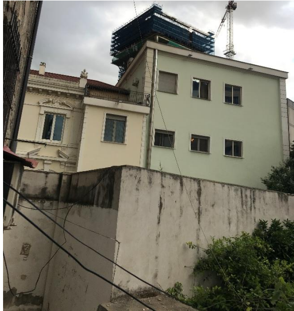
Figure 284. Front entry surrounded by walls (6)
