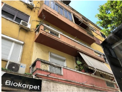
Figure 253. Balcony typology on the site (2)
