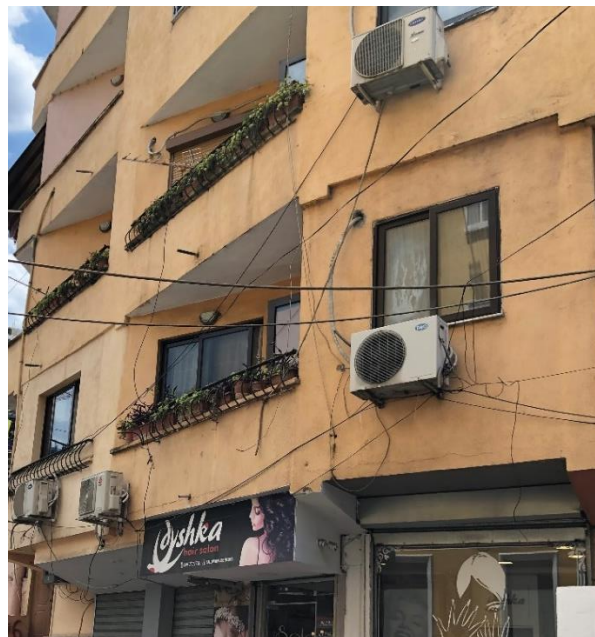
Figure 269. Balcony typology on the site (19)
